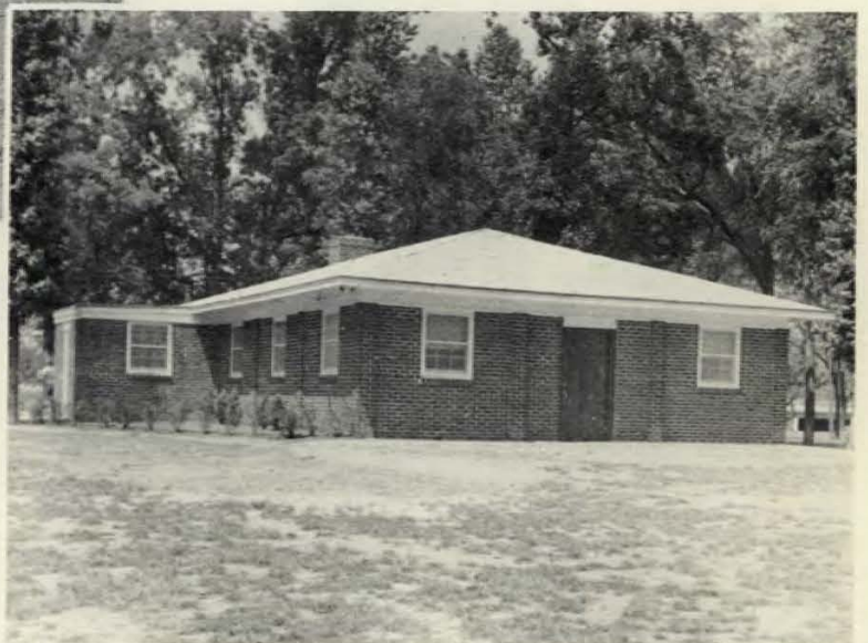
The Lane Manor Recreation Center in Northwest Branch Park is shown as it was under construction in February, 1956, as an open type shelter. When funds became available last year, the Commission enclosed the building to enable maximum community use of the facility.
