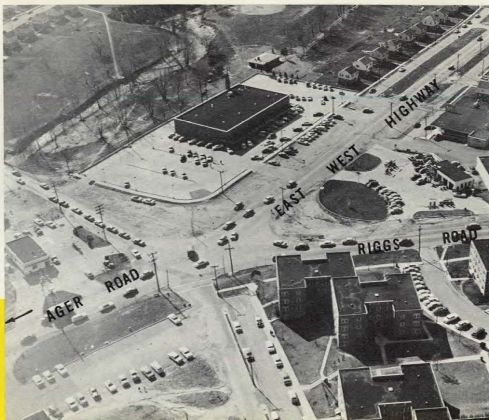
The Commission's proposal for channelization of traffic at the Riggs Road-East West Highway intersection in Prince George's County is shown in a sketch above. The accompanying photo illustrates the problem at the busy intersection because of the five-way movements of traffic.
