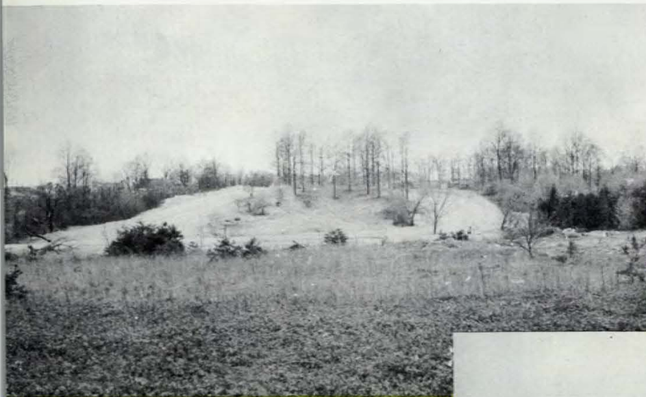
Preliminary grading foretells the development of a new subdivision.
