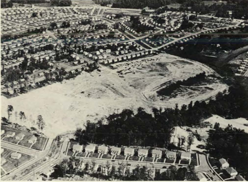
THE PHOTOGRAPHS on these two pages show how the population of the area under the Commission's jurisdiction is steadily increasing. This picture of a subdivision being developed just west of Georgia Avenue in Glenmont was taken about a year ago.
