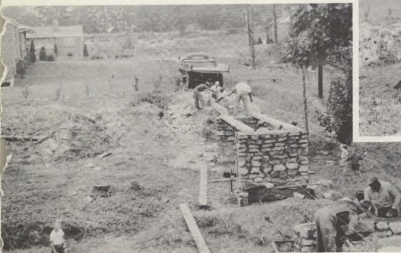
Another bridge goes up in Long Branch Park.
