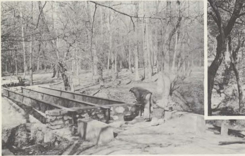
Bridge under construction across Rock Creek.
