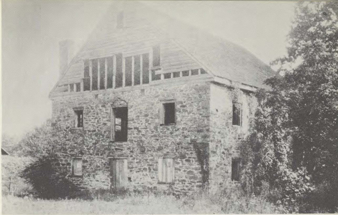
This is how the mill looked when the Commission acquired it in 1951. It was once owned by the Riggs family for whom Riggs Road was named.
