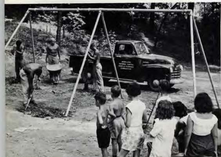
After the park is cleared, Commission workers install play equipment.
