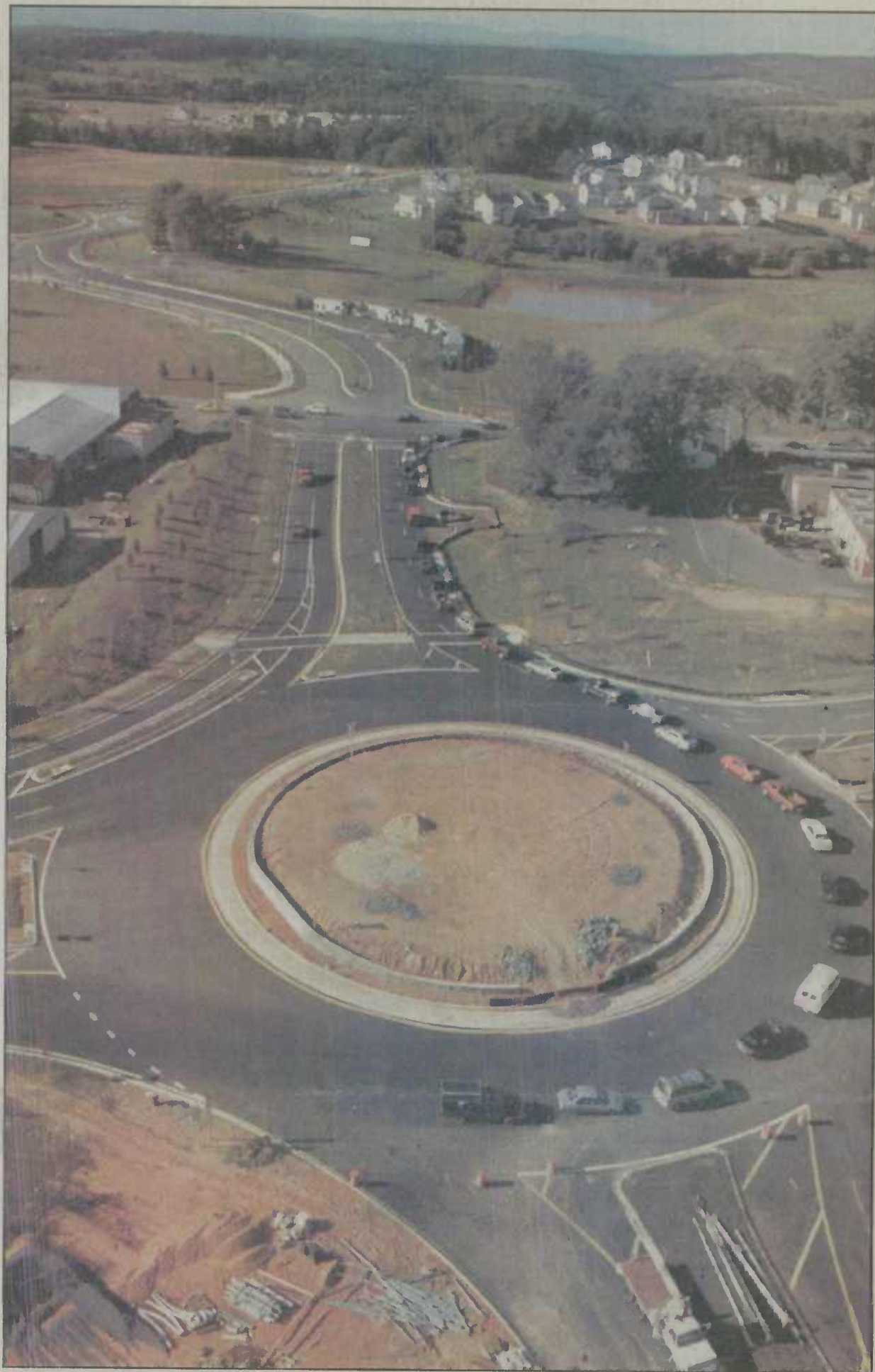
80 The newly completed traffic rotary in Urbana connects I-270, Md. 85 and Md. 355.
