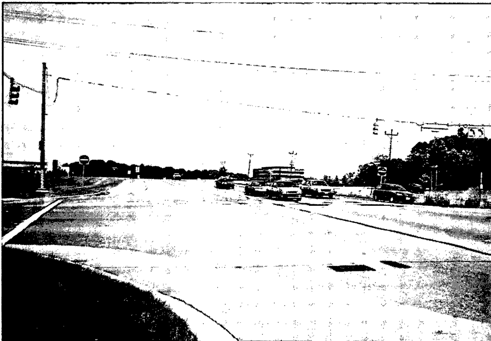
VI. Tech Road - Just southwest of intersection looking north.
