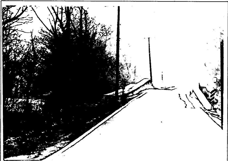
PHOTO 4—Devil's Backbone Bridge: Poor road width couple with poor visual sighting.
