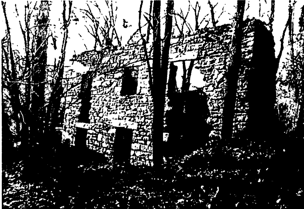
Photograph 22: South Wall of Mill in 1989
