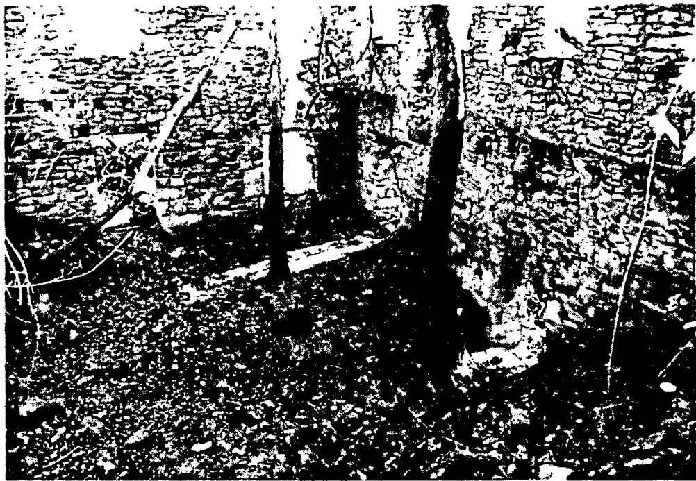
Photograph 7: View Inside Mill (F1). Note Large Trees in Center
