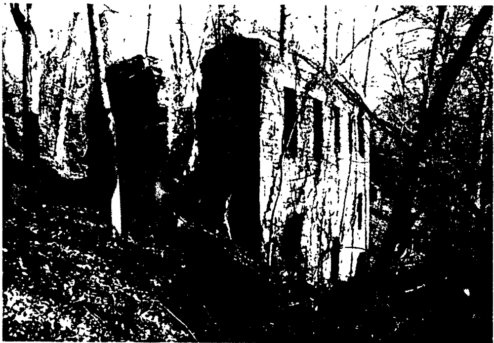
Photograph 15: View of Northwest Corner of Mill in 1989
