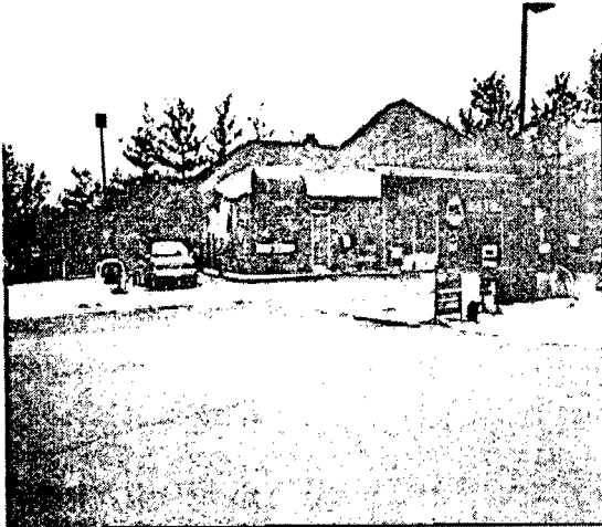
Mobile Service Station
