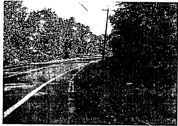
looking eastward along MD 28, east of MD 97
