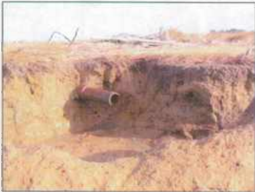
Exposed pipe at low tide on northern shoreline of Northern Remnant
