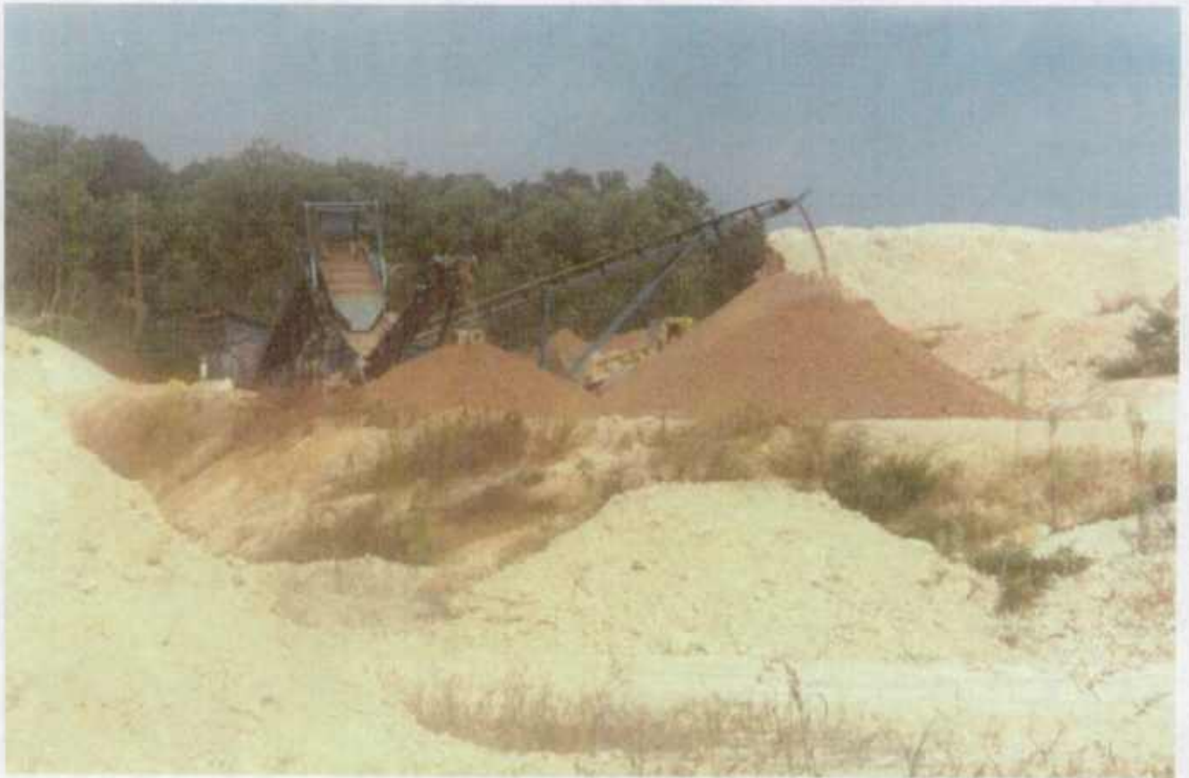
Figure 3.5 – Clay Material For The Cecil County Landfill
