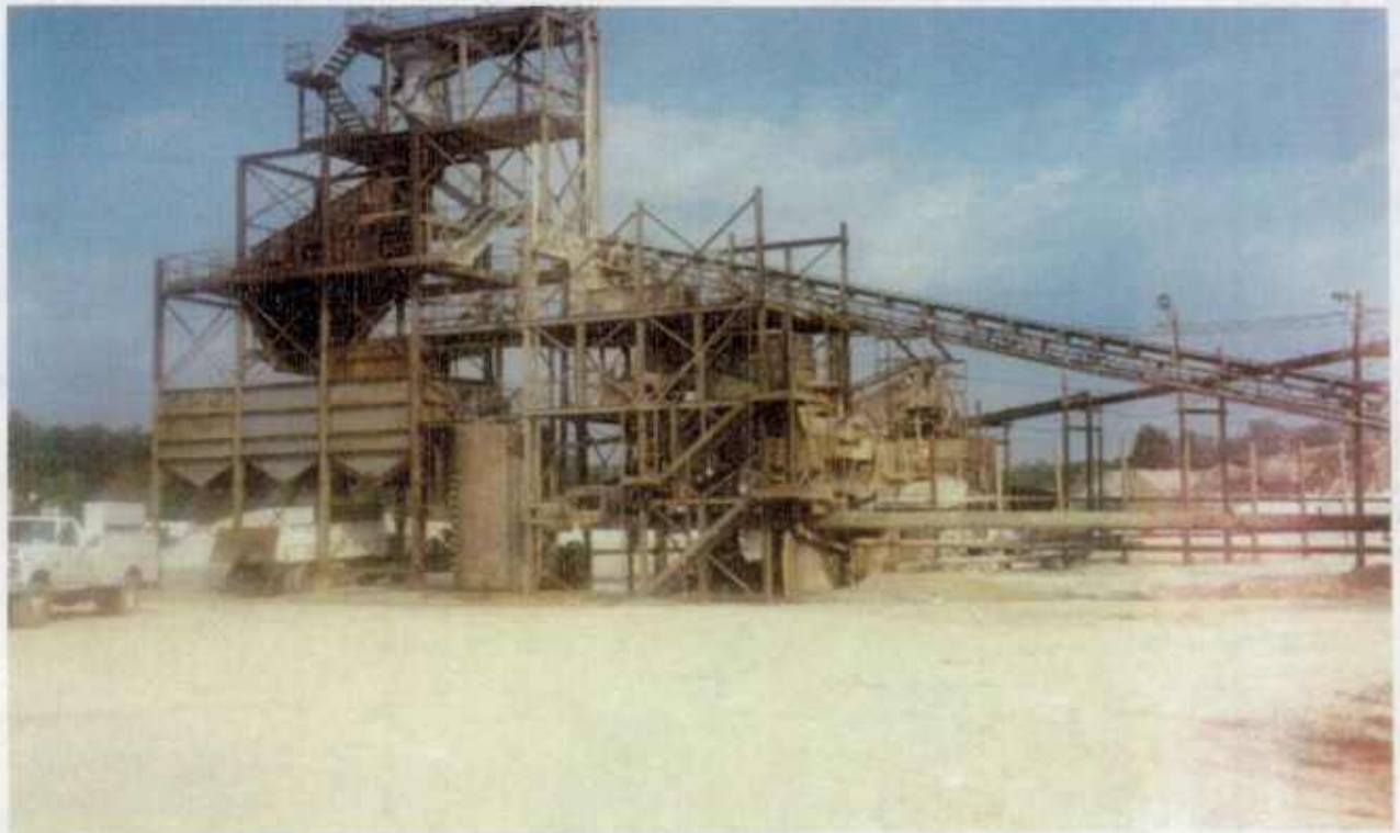
Figure 3.2 – Washing and Grading Facilities
