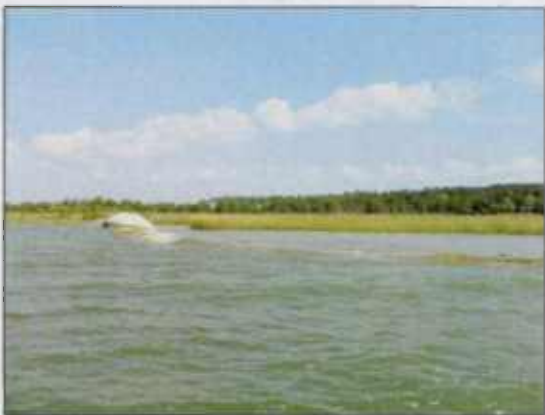
Looking northeast at geotubes adjacent to created wetland.
