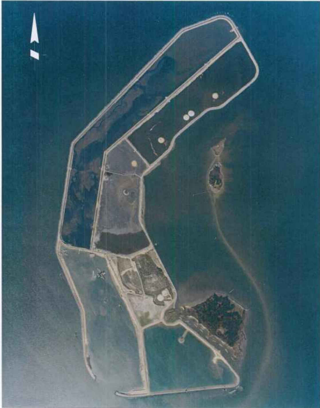
Figure 2-2: Poplar Island Environmental Restoration Project November 2001 Aerial Photograph
