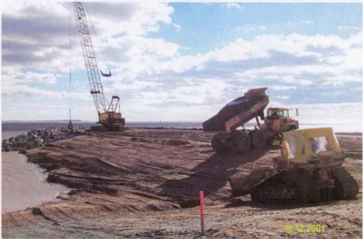
George and Lynch Grading Dike Fill SW Cell 6 December 2001
