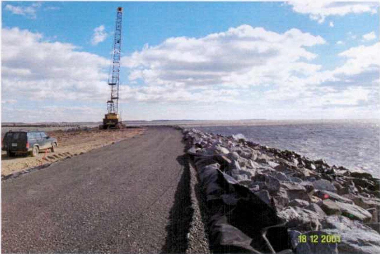
Completed Slope Stone and Roadway - West Cell 6 December 2001
