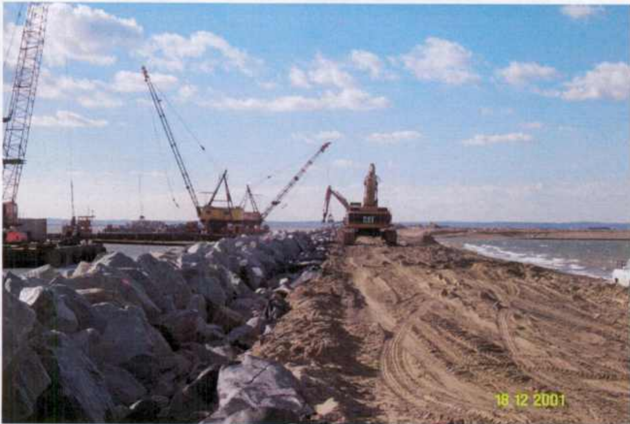
Tidewater Placing Slope Stone on South Dike December 2001
