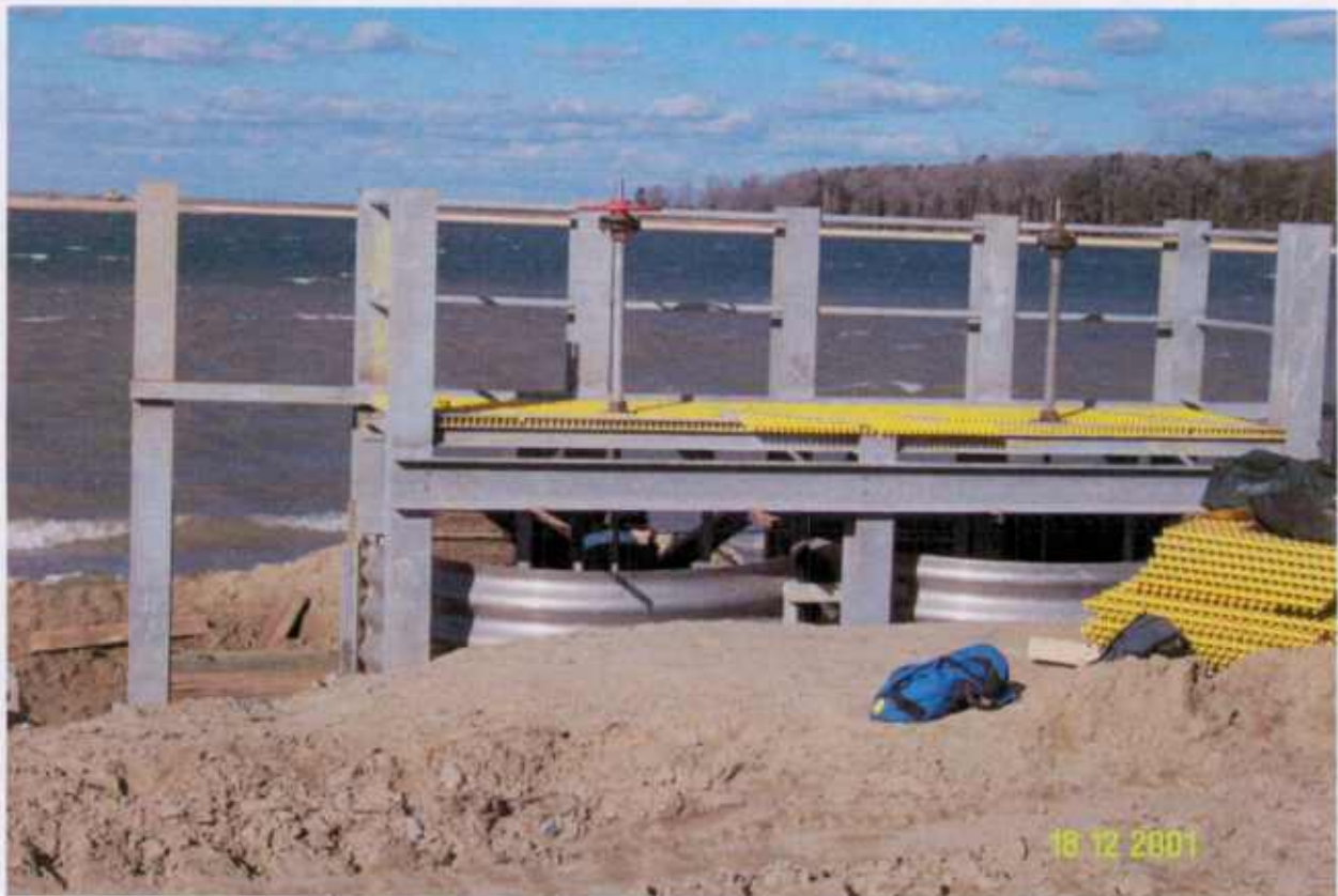
Spillway Installation – Cell 5 December 2001
