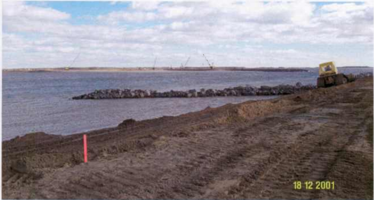
George and Lynch Grading Dike Fill SW Cell 6 December 2001
