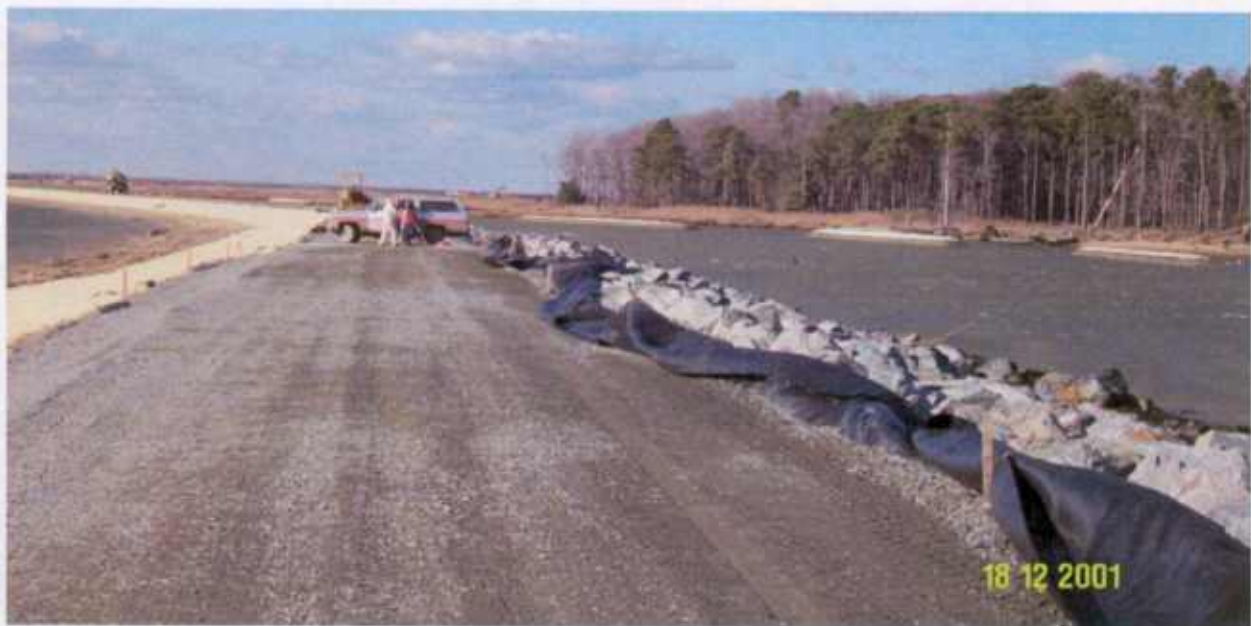
Completed Slope Stone and Roadway - East Cell 6 December 2001
