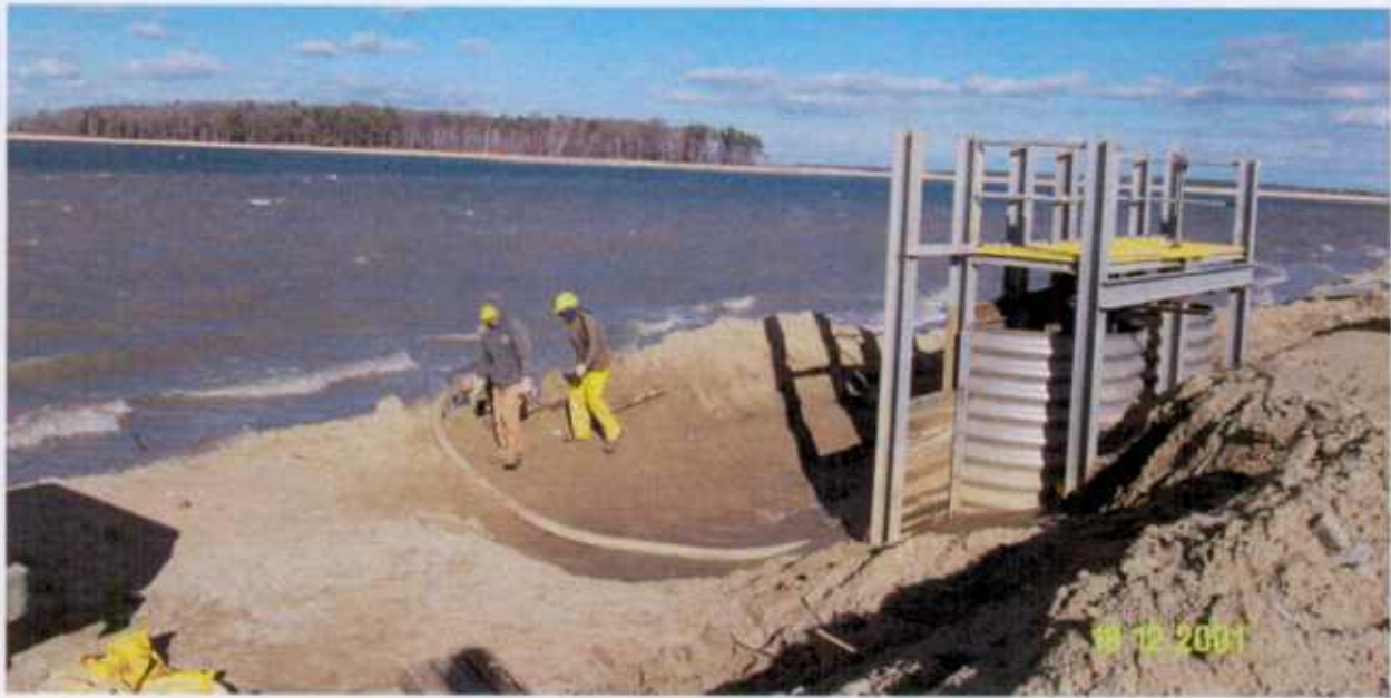
Spillway Installation – Cell 5 December 2001
