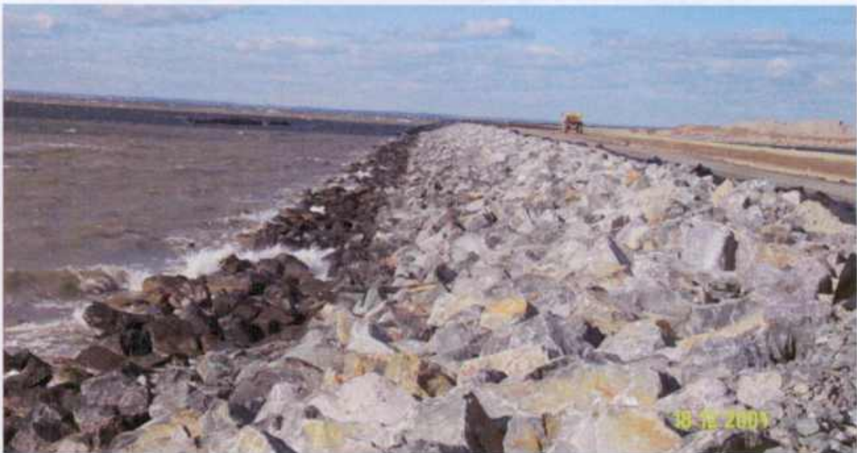
Completed Slope Stone and Roadway - West Cell 6 December 2001
