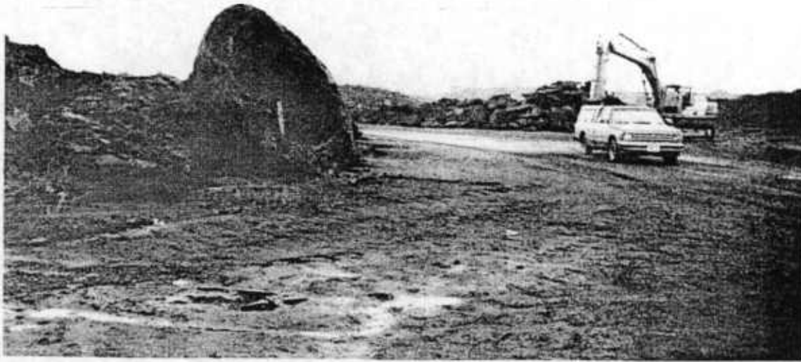
View of Slag Piles at Surface (near El +10±) Note "SKULL" in the foreground
