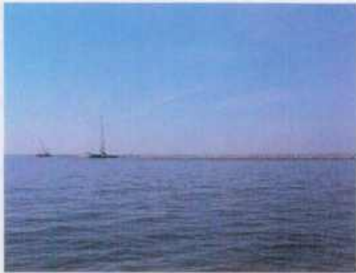
Poplar Island – Modification P14. Looking west towards Poplar dike at the construction of Phase II.
