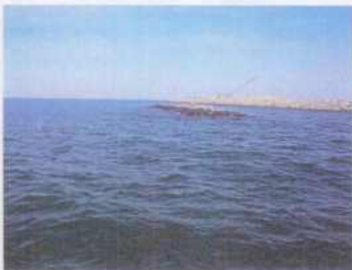
Poplar Island – Modification P1. Looking north towards dike from benthic monitoring site 005.
