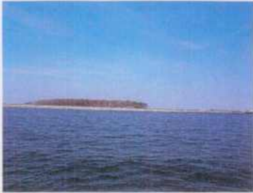
Poplar Island – Modification P22. Looking north at riprap on southern dike on Poplar and Coaches Islands from benthic monitoring site 010.
