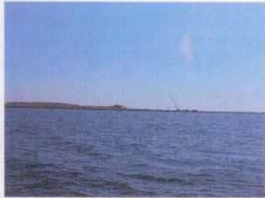
Poplar Island – Modification P3. Sitting near the edge of the dike for modification looking to an area of potential modification on the west side of the island.
