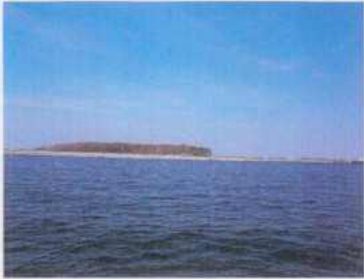
Poplar Island – Modification P22. Looking north at riprap on southern dike on Poplar and Coaches Islands from benthic monitoring site 010.
