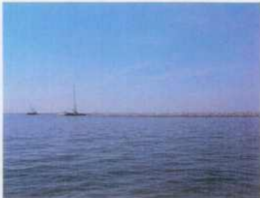
Poplar Island – Modification P14. Looking west towards Poplar dike at the construction of Phase II.
