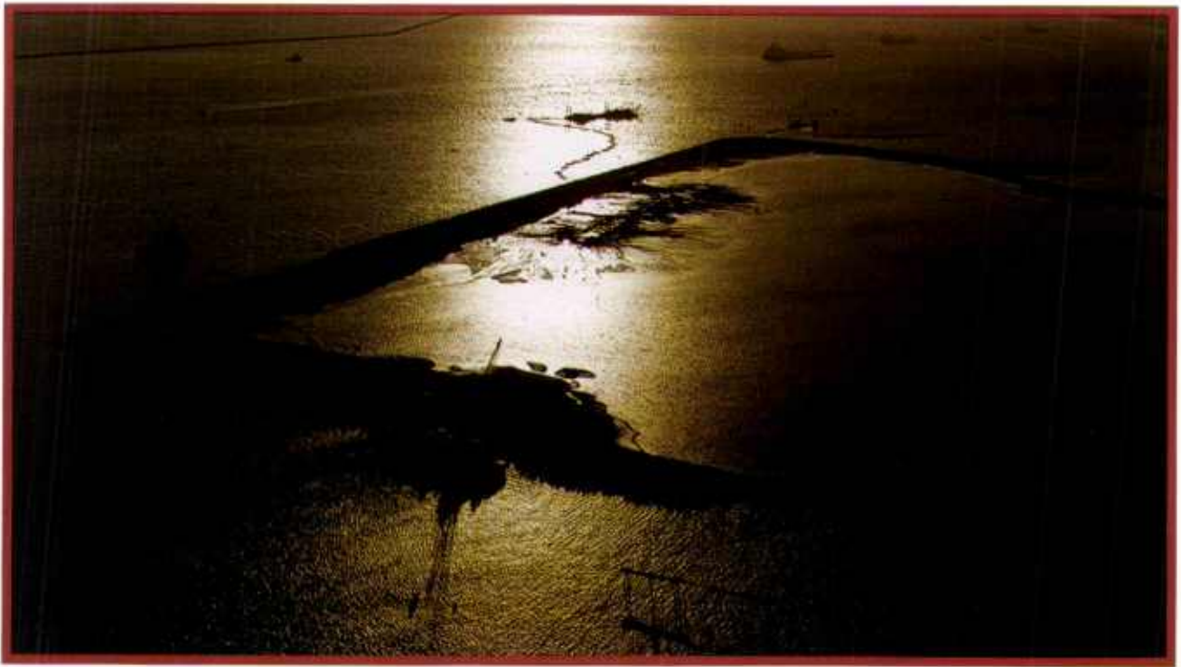
Pier Expansion: The Florida is visible on the far side of the emerging land mass of Pier J in Long Beach, California. The electric-powered Florida pumped the fill for this 120-acre (48-hectare) expansion program.
