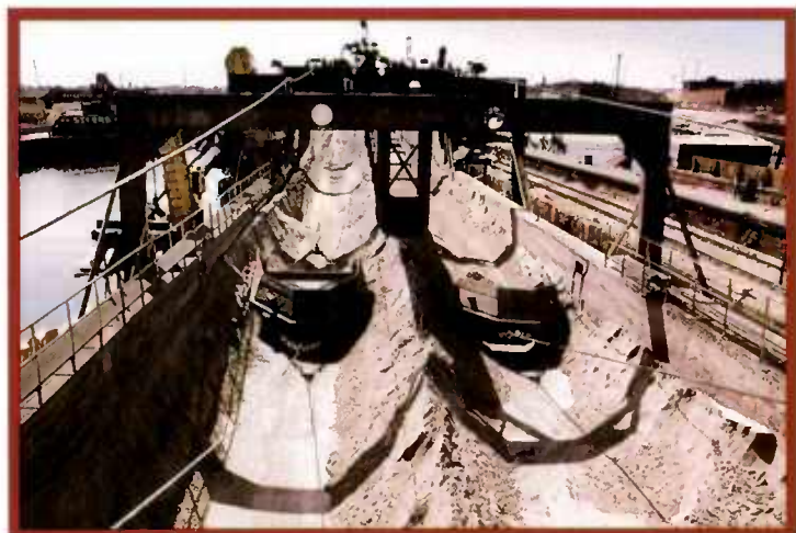
Material Transfer: The Sandy Hook nears the Amboy Aggregates dock with a load of material (above). Unloading is facilitated by a bucket system that feeds a shoreside conveyor.
