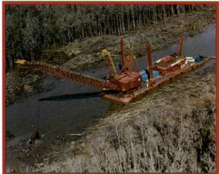
A 200-foot boom suits Dredge No. 54 for long side-casting jobs.
