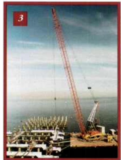
Deck Work Under Way: The trestle and pier measure 2,445 feet (745 m) in extent. (1) (Below) The crane on the jack-up barge raises a pile for driving. (2) Positioning a pile cap. (3) Barge-mounted 4100 Ringer Crane lifts caps into position; boom length is 230 ft.
