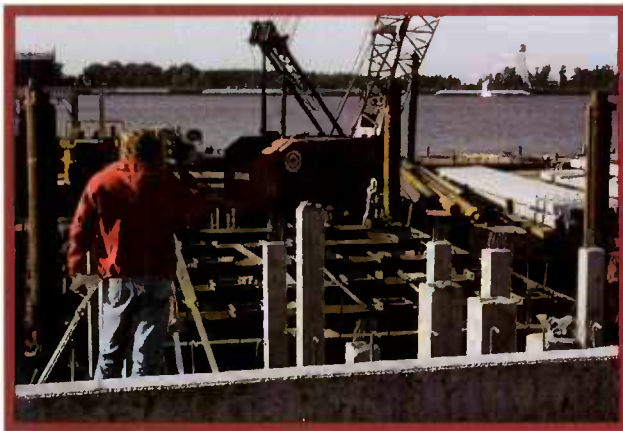
Pile driver nears completion of a section of steel pilings. Below left, final adjustments of the template are made. Below right, steel pilings have been cut off at deck level. The tight construction schedule called for commencement of driving operations 45 days after contract award.
