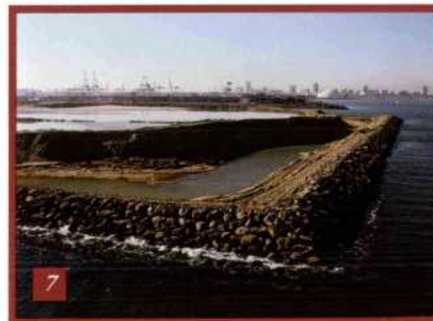
Fill Management: 5) Bulldozers working the fill at the discharge of Florida's pipeline. 6) Reclamation area as Lift 6 emerges from the water. 7) Water level "A" rock is in place, with surcharge under construction. 8) Project nearing completion.
