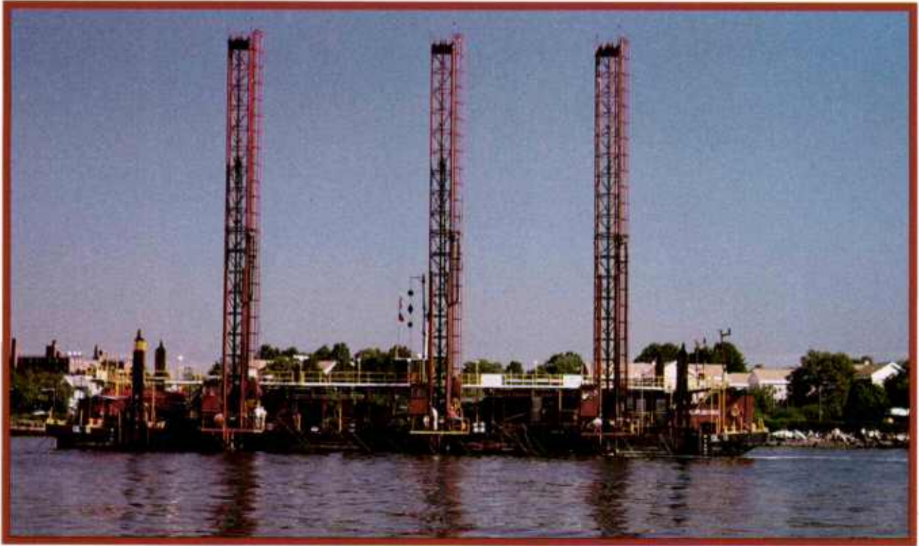
Drillboat No. 8 in New York Harbor: Two Great Lakes drillboats worked on the deepening of the Kill Van Kull, the largest dredging project in the history of the U.S. Army Corps of Engineers. The project required drilling and placement of more than 150,000 charges.
