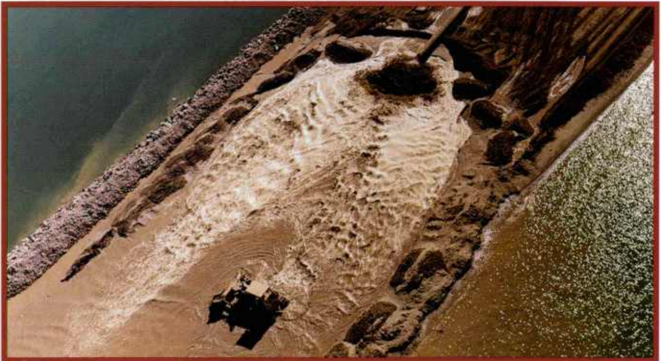
Dredging & Filling: Portions of the fill were along narrow sections of the lining of the facility. Below, left, Dredge No. 53 removed unsuitable material from under the rock perimeter wall. At right, a clay material cutterhead of the dredge Florida.
