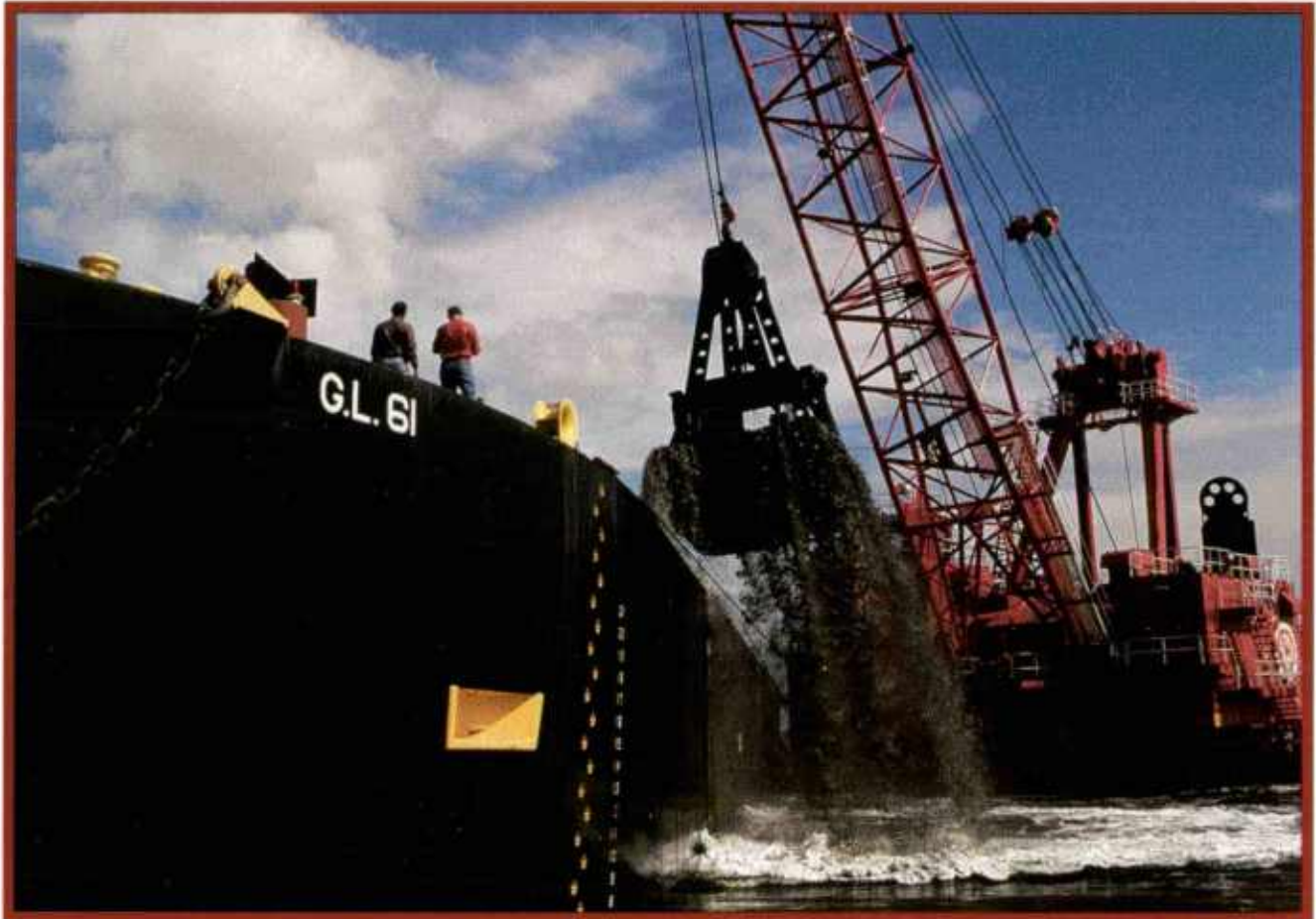
The dredge Chicago, the largest bucket dredge in the Great Lakes fleet, reflects the company's commitment to design and construction of the finest dredging equipment. She is the most efficient clamshell (grab)dipper dredge in the world.
