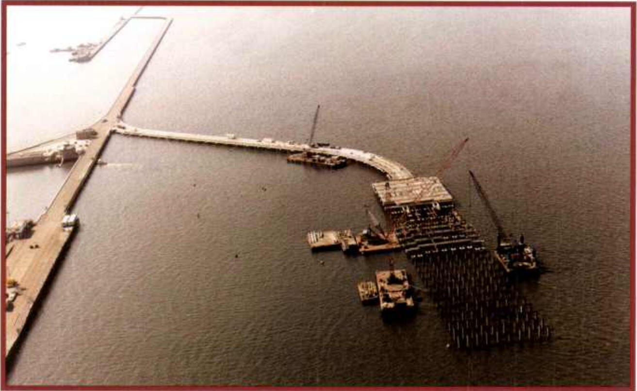
Deck Work Under Way: The trestle and pier measure 2,445 feet (745 m) in extent. (1) (Below) The crane on the jack-up barge raises a pile for driving. (2) Positioning a pile cap. (3) Barge-mounted 4100 Ringer Crane lifts caps into position; boom length is 230 ft.
