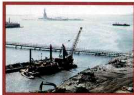
The trailing suction hopper dredge Northerly Island (above) transports material for placement. At right above, the hydraulic cutterhead dredge Georgia excavated silts and sand on the project. Below right, clamshell Dredge No. 50 removes material preparatory to placement of fill and armor stone.
