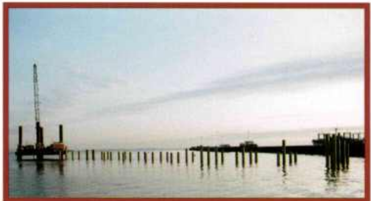
Ammunition Pier: Finished and in operation. Below, pile-driving proceeds from the deck of a jack-up barge. At bottom, precast, prestressed concrete caps are positioned atop the pilings.
