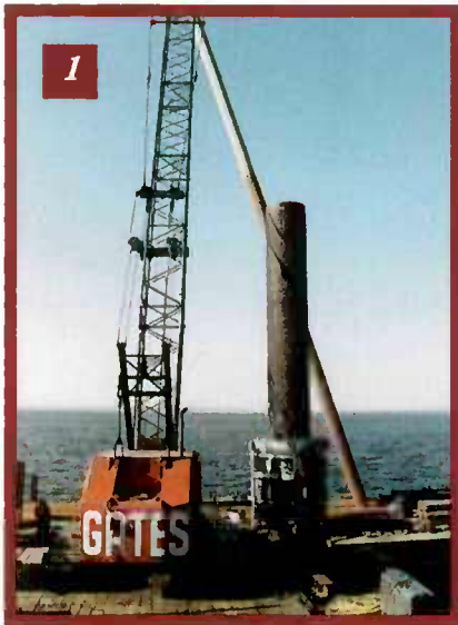
Deck Work Under Way: The trestle and pier measure 2,445 feet (745 m) in extent. (1) (Below) The crane on the jack-up barge raises a pile for driving. (2) Positioning a pile cap. (3) Barge-mounted 4100 Ringer Crane lifts caps into position; boom length is 230 ft.
