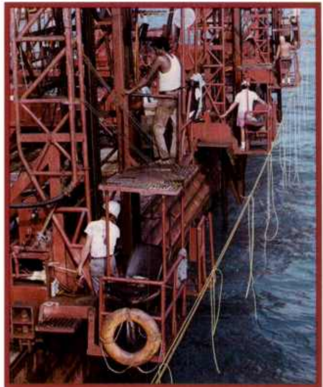
In dipper mode, the dredge Boston digs in the entrance channel to Jebel Ali (above). Below left, the hydraulic cutterhead dredge Georgia; at right, workers on the drillboat Algonquin rig holes drilled in the rock for blasting.
