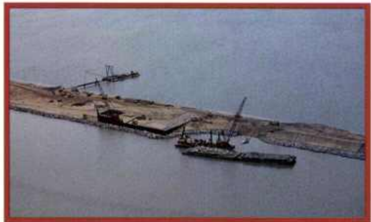
The completed containment area at Hart-Miller Island. Below, a crane prepares to offload roadbed material. At bottom, a Gradall begins dressing foundation stone laid on top of filter cloth.
