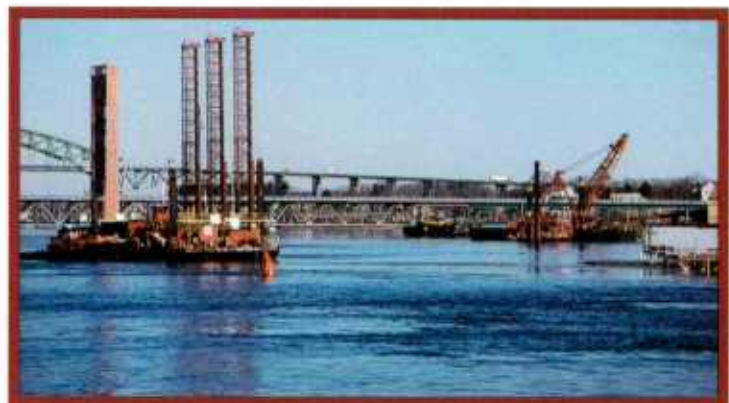
Drilling & Blasting: The convertible clamshell/dipper dredge Boston, in clamshell mode, dug material blasted by Drillboat No. 8, below.
