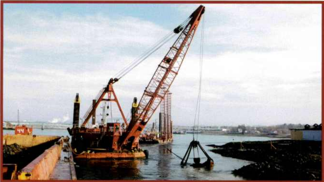
Drilling & Blasting: The convertible clamshell/dipper dredge Boston, in clamshell mode, dug material blasted by Drillboat No. 8, below.
