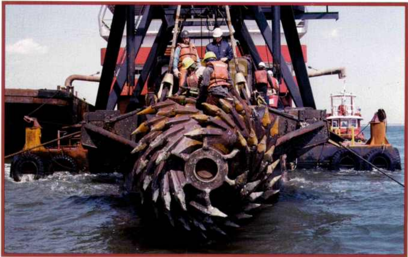
Rock Cutter: The Carolina routinely excavates unblasted rock.
