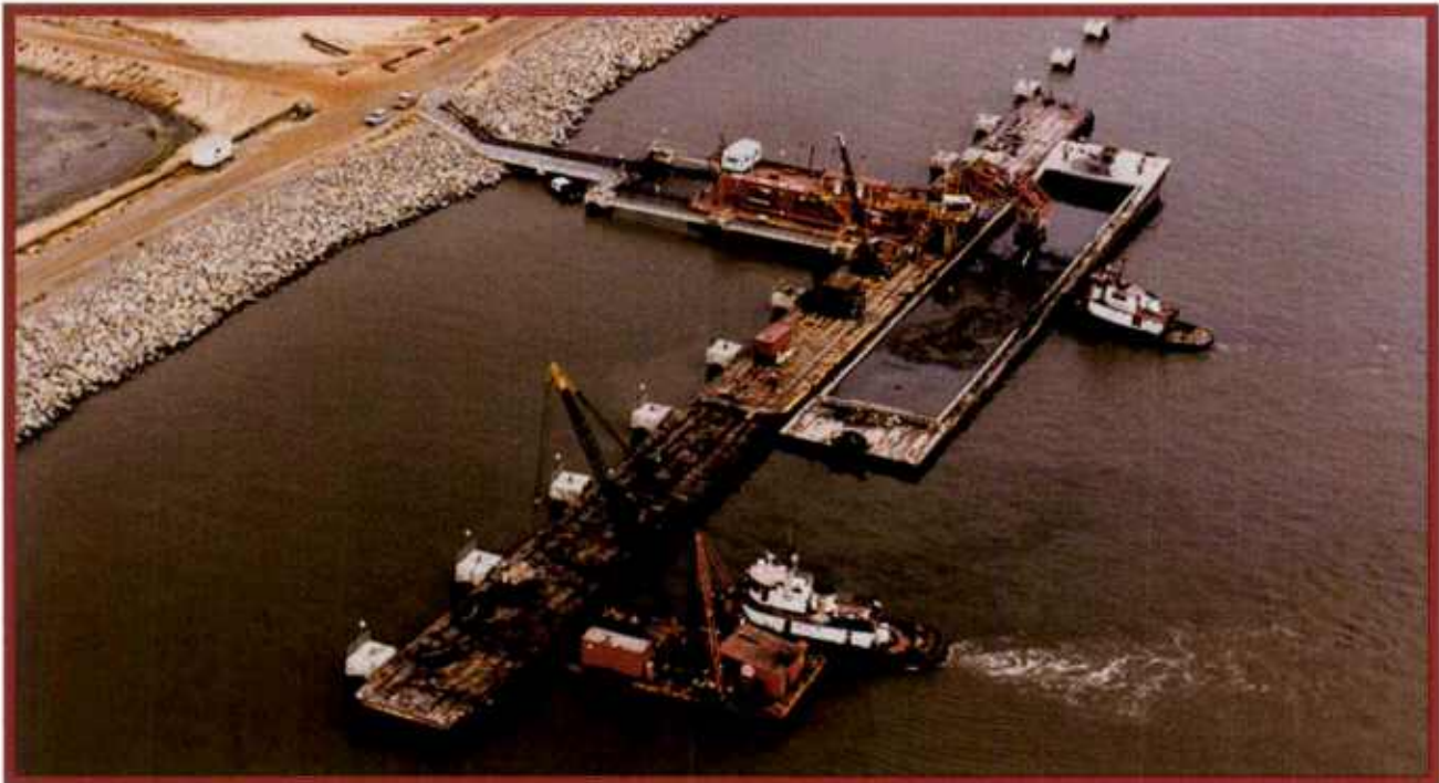
Facility Layout: Since its construction, Great Lakes has placed more than 44,000,000 yd 3 (33,640,000 m 3 ) in the containment facility. Below, hydraulic Unloader No. 2 pumps material from a barge at the south unloading facility.
