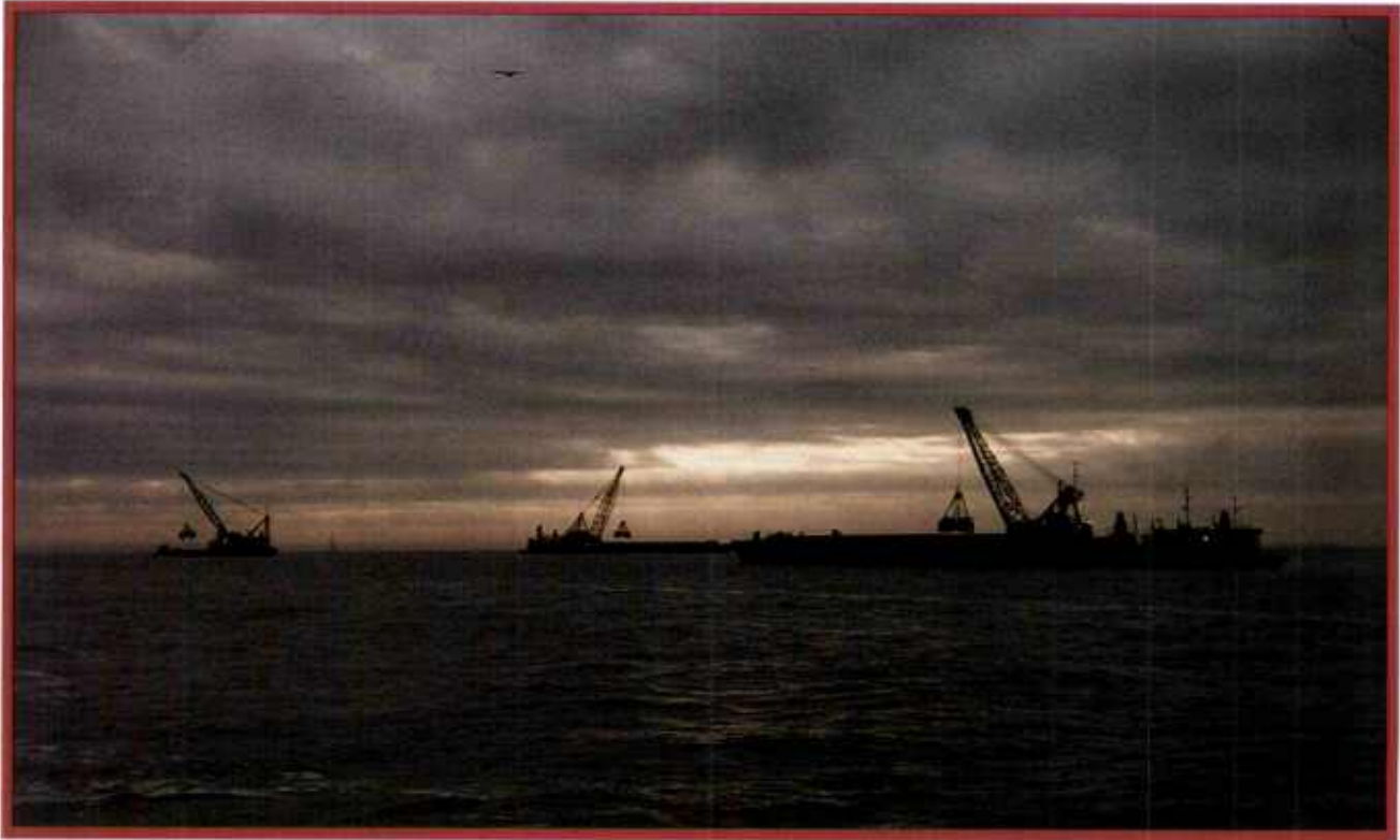
Great Lakes Clamshell Dredges No. 50, 51 and 52 at work deepening the approach channels to Baltimore Harbor.
