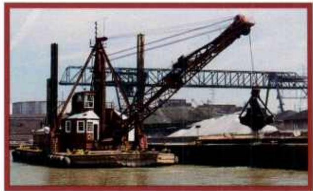
Dredge No. 55 performs riverfront maintenance dredging.
