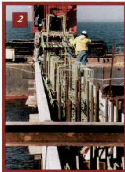
Deck Work Under Way: The trestle and pier measure 2,445 feet (745 m) in extent. (1) (Below) The crane on the jack-up barge raises a pile for driving. (2) Positioning a pile cap. (3) Barge-mounted 4100 Ringer Crane lifts caps into position; boom length is 230 ft.
