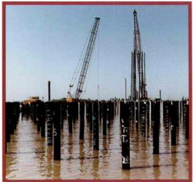
Pile driver nears completion of a section of steel pilings. Below left, final adjustments of the template are made. Below right, steel pilings have been cut off at deck level. The tight construction schedule called for commencement of driving operations 45 days after contract award.
