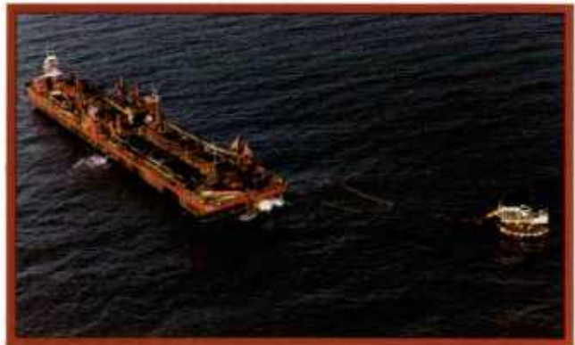
Offshore dredging for Phase I was performed by the hydraulic cutterhead dredge Carolina (above) and the trailing suction hopper dredge Long Island, shown pumping material ashore via the SCOTS Buoy.
