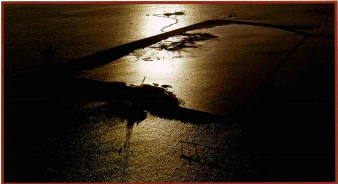
Pier J in Progress: The dredge Florida (visible at top center) pumps sand into the main fill. Below, after completion of the project, the 120-acre (50-hectare) plot undergoes development. At bottom, the Florida at work early in the project.
