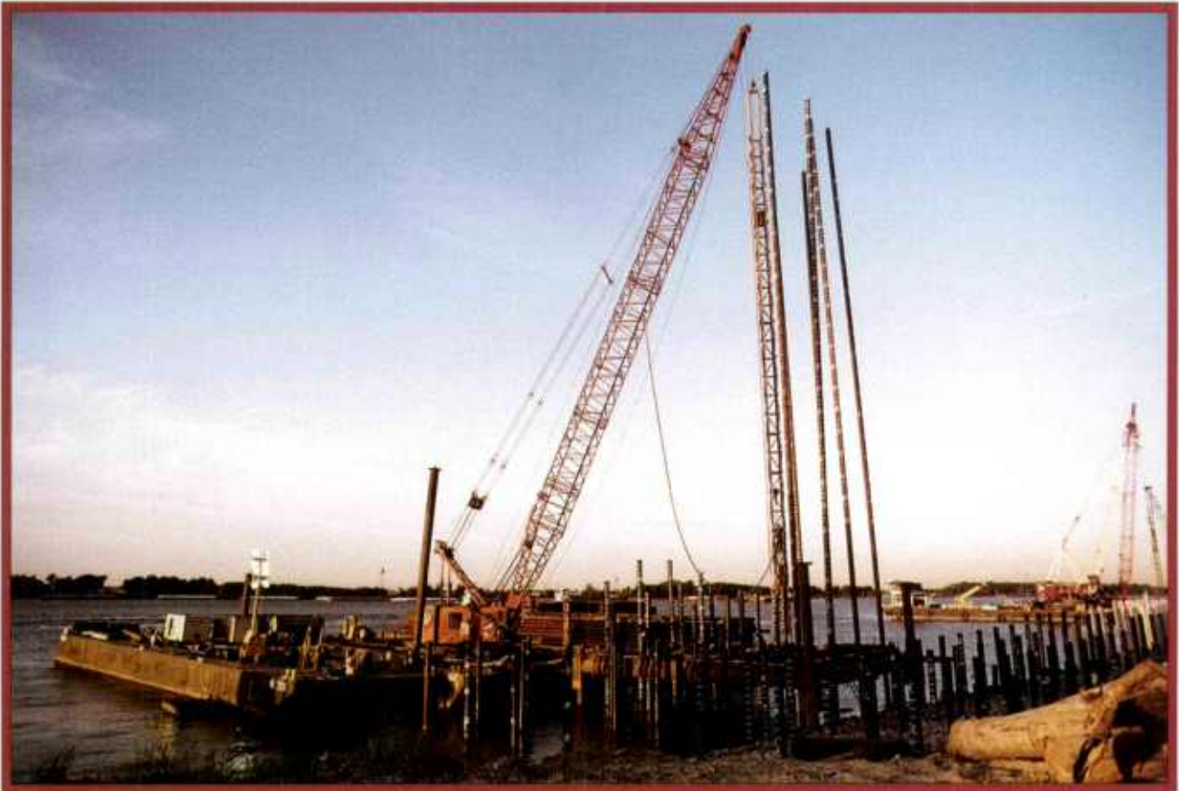
Pile driver nears completion of a section of steel pilings. Below left, final adjustments of the template are made. Below right, steel pilings have been cut off at deck level. The tight construction schedule called for commencement of driving operations 45 days after contract award.
