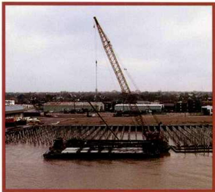
Crane removes a tubular steel pile from barge for placement.
