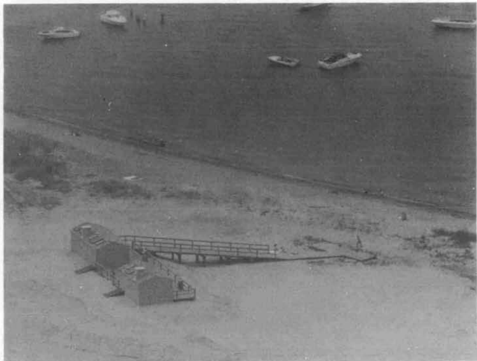
Clivus Restroom Buildings, Hart-Miller Island State Park, Chesapeake Bay (near Baltimore) -- Heavy use with no discharge.
