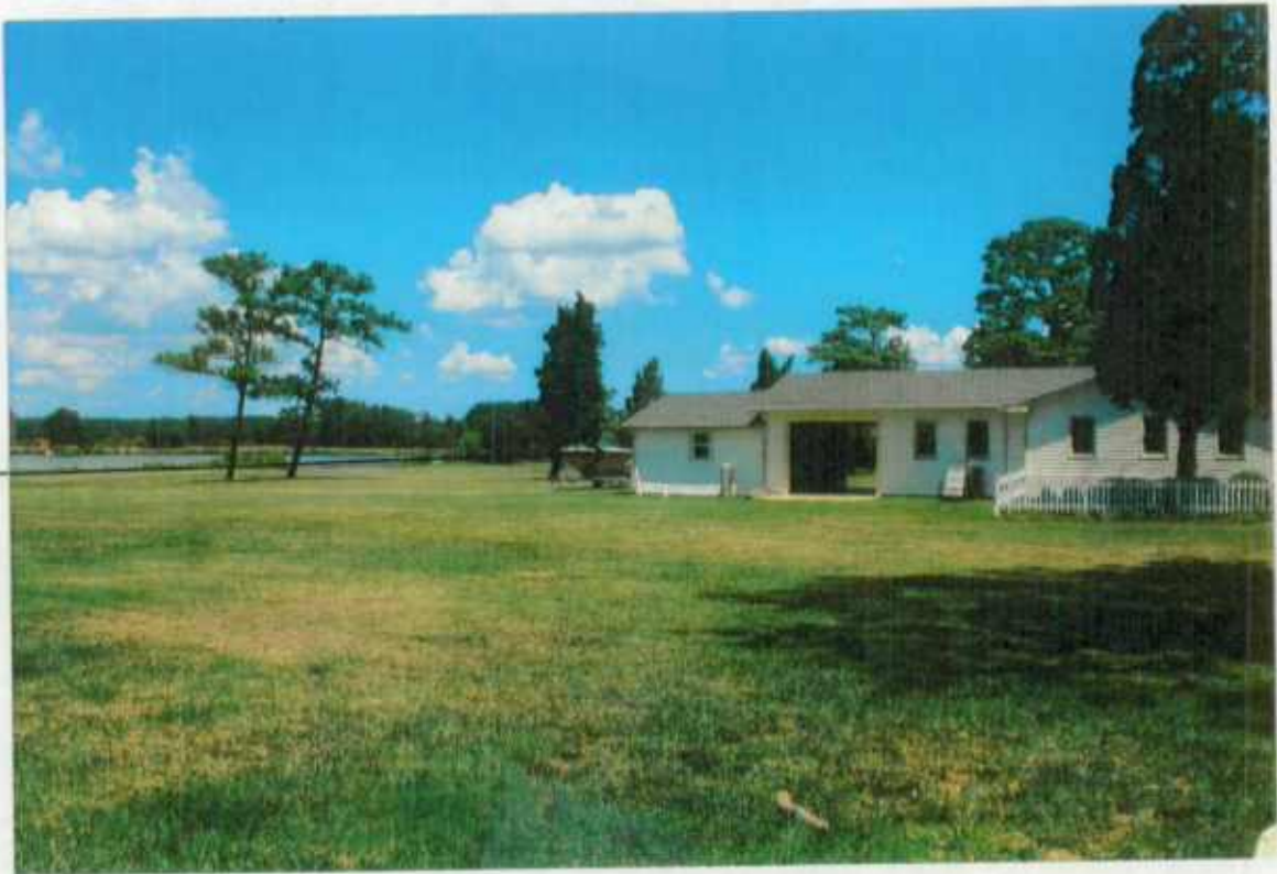
Neighbor #2 ancillary structure in Buffer
