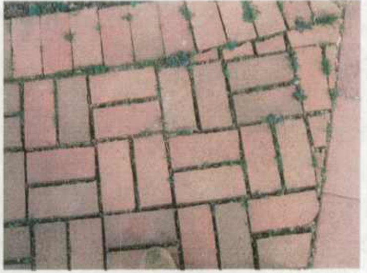
Brick Walk ON Sand Bed
