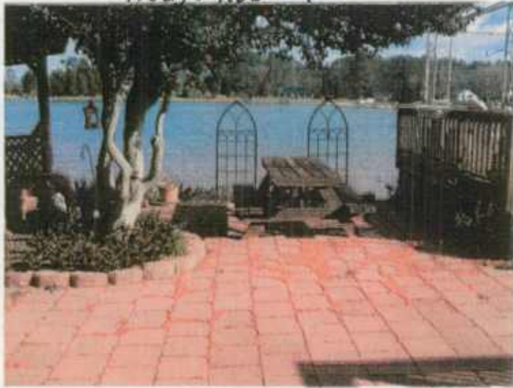
Brick Pad on Sand Bed.
