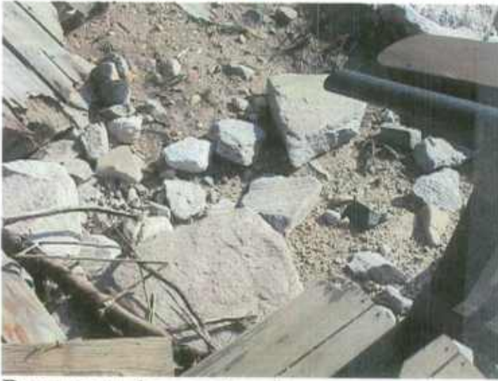
Revetment damaged again
