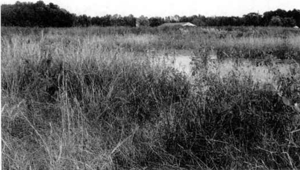
Photo 31 3909 Ponding in Phase I Oct 2009
