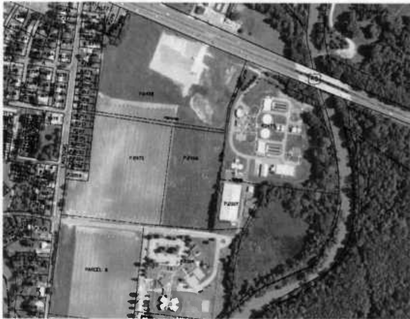
Aerial view of existing WWTP and the expansion site
