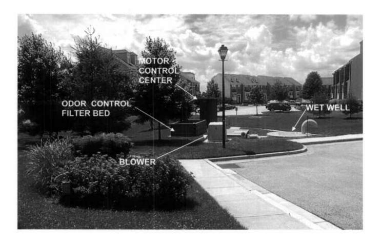
The pump station would be constructed on the East side of and adjacent to the existing tennis court and is designed to have a low profile and small footprint. The SPS will be mostly underground except for a motor control center and a back up generator. The motor control center
