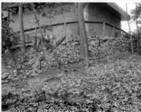
Neighboring home/erosion control
