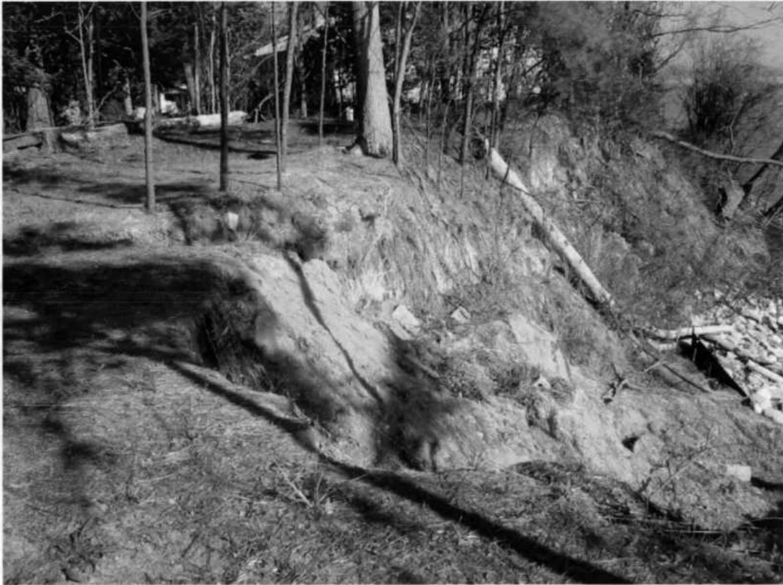
White Property-Cliff Collapse 1/3/05
