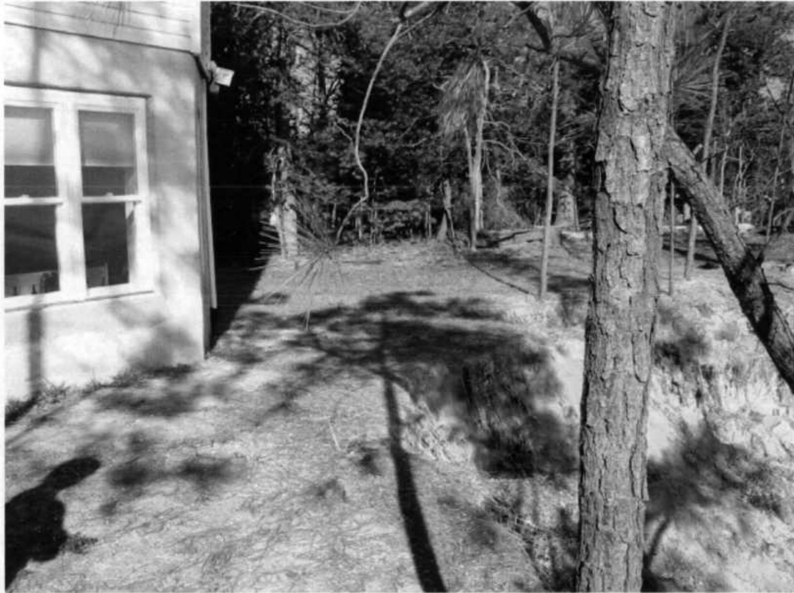
White Property-Cliff Collapse 1/3/05
