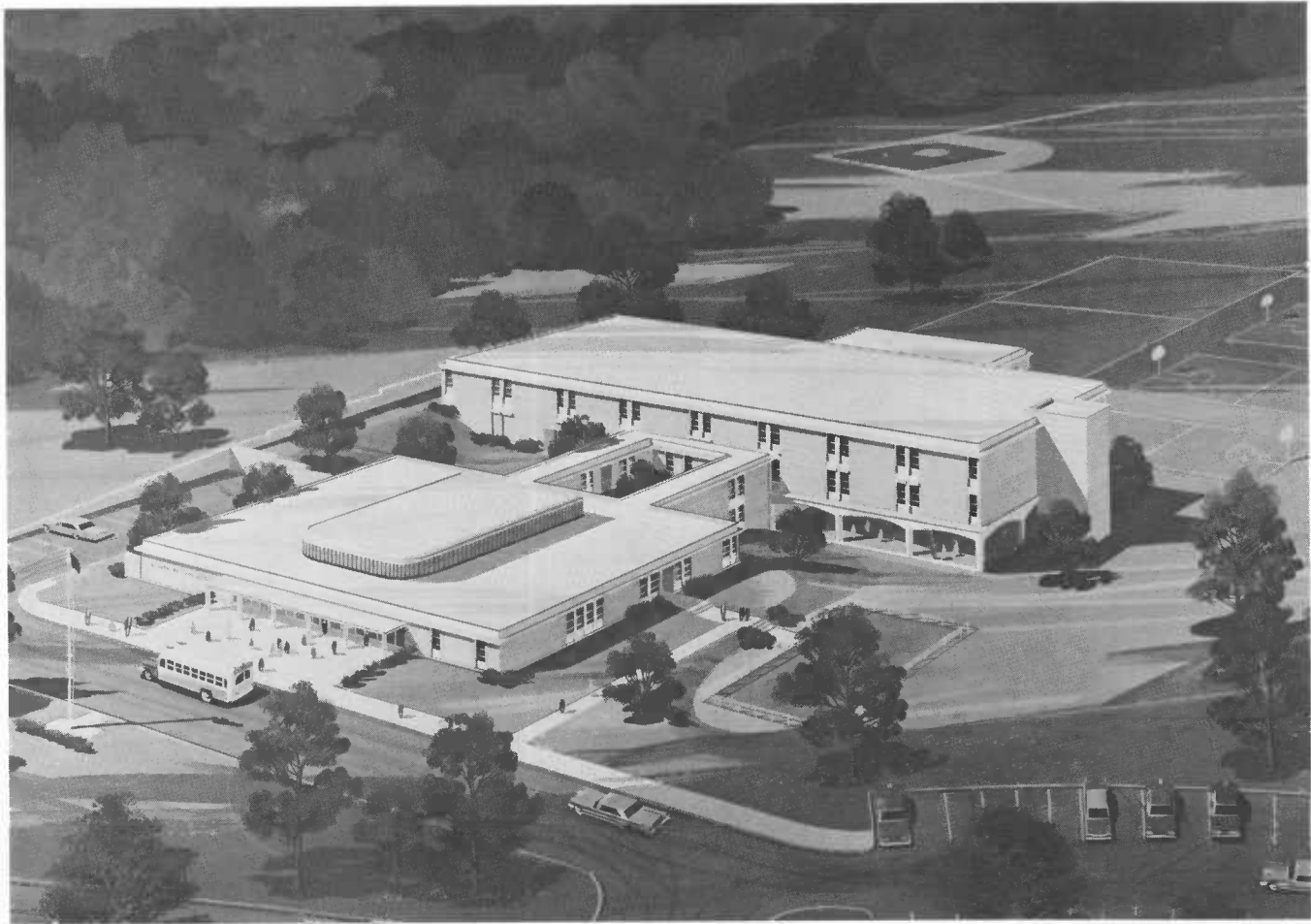
The Templeton Manor Elementary School is tentatively scheduled for completion in the fall of 1968. The school will include 20 regular classrooms, 2 kindergarten rooms, 2 special education rooms, and a gymnasium. The construction cost is $1,240,000.
