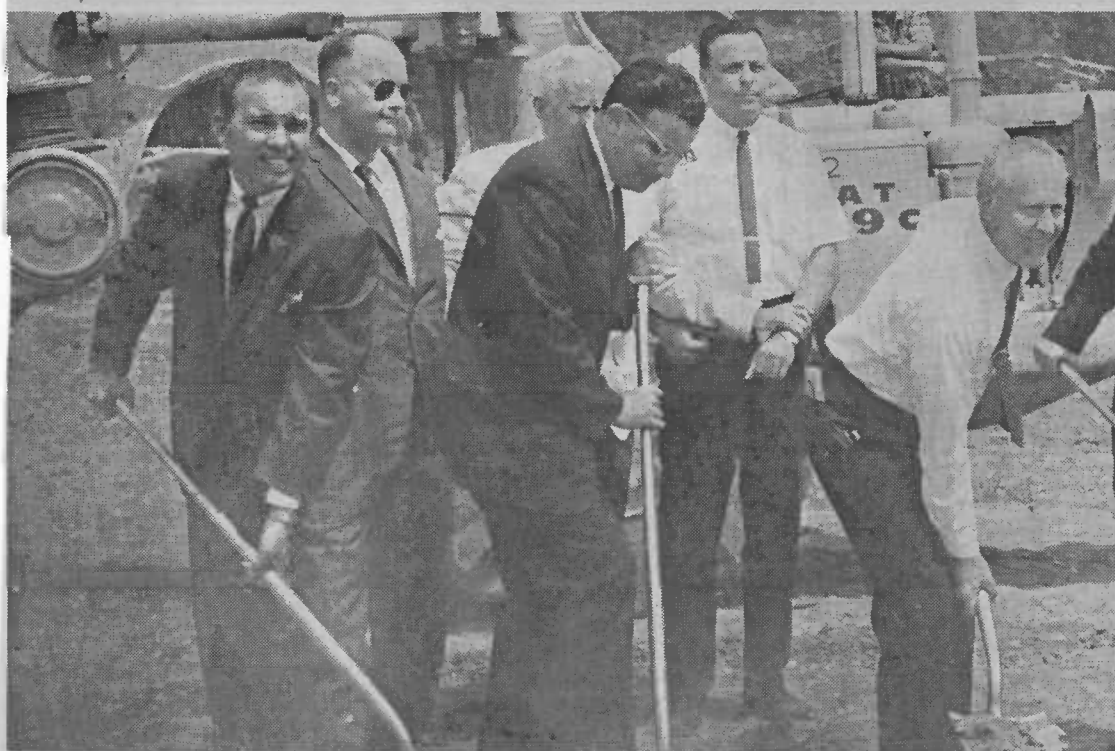
DIGGING IN FOR PRINCE GEORGES—Wielding shovels at groundbreaking ceremony for new State Roads Commission Building at Greenbelt are (left to right) State Senator Fred L. Wineland (D., Prince Georges), Delegate Arthur Dorman, William C. Birely, of the Montgomery County Council, and Comptroller Louis Goldstein. The $780,000 building will be erected on a site at the intersection of the Capital Beltway (Interstate 495) and Kenilworth Avenue (Route 201).
