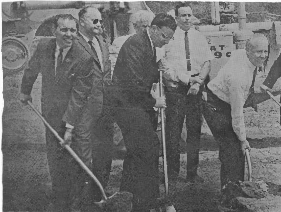
GROUND BREAKING--Bringing construction work to a start for the new State Roads Commission Building at Greenbelt are State Senator Fred L. Winland (D. Prince Georges), William C. Birely, of the Montgomery County Council, and Comptroller Louis Goldstein. The $780,000 building will be erected on a site at the intersection of the Capital Beltway (Interstate 495) and Kenilworth Ave. (Route 201)
