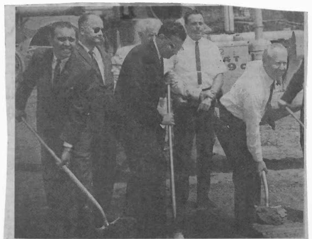
DIGGING IN FOR PRINCE GEORGES - Wielding shovels at ground-breaking ceremony for new State Roads Commission Building at Greenbelt are (left to right) State Senator Fred L. Wineland, (D., Prince Georges), Dr. Arthur Dorman, Prince Georges Delegate (D), and Comptroller Louis Goldstein. The $780,000 building will be erected on a site at the intersection of the Capital Beltway (Interstate 495) and Kenilworth Avenue (Route 201).
