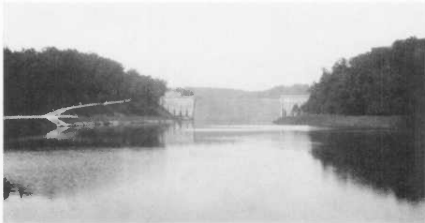
Fig. 1. Gunpowder Falls below Loch Raven Dam
