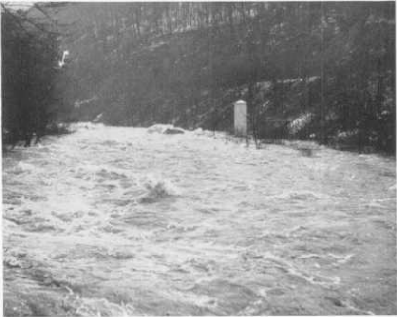
FIGURE 1. Gage house on Savage River below Savage River Dam after releasing about 5,000 cfs at dam.
