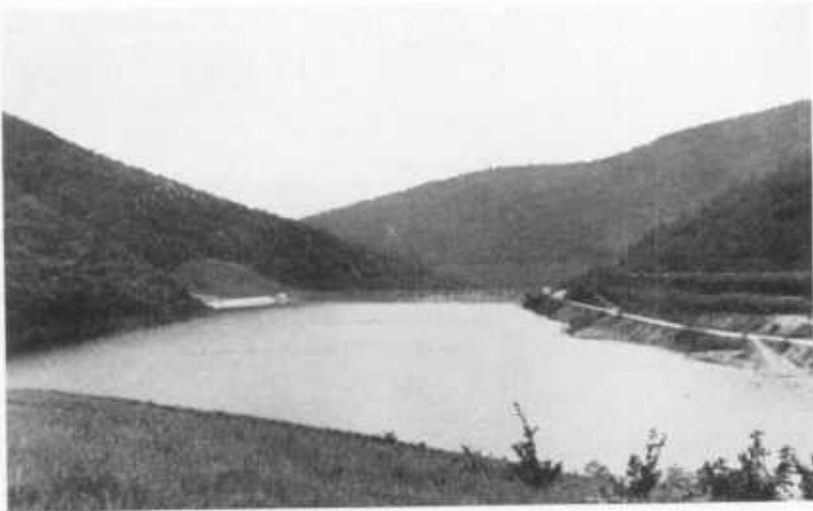
FIGURE 2. Savage River Dam showing spillway on left side.
