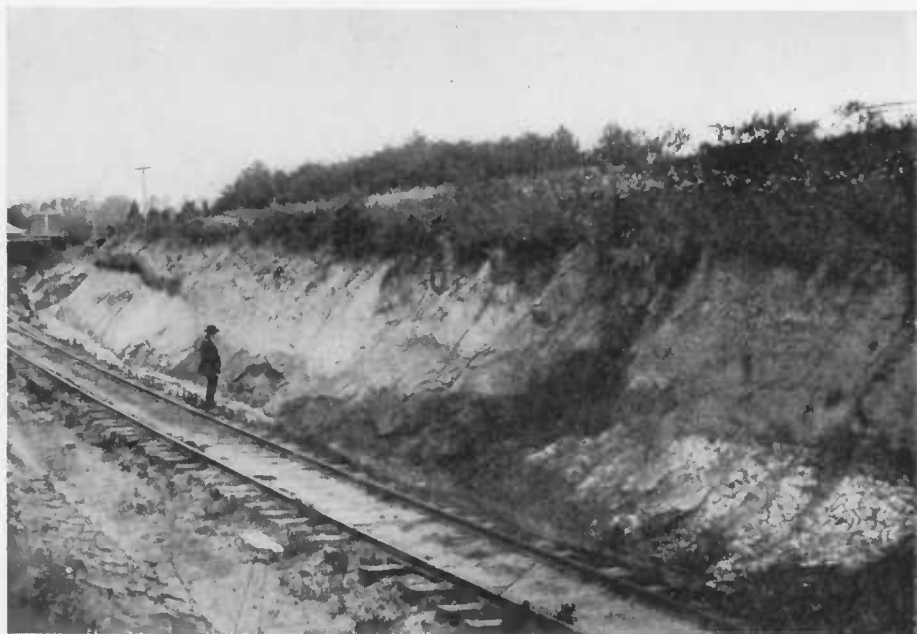
FIG. 2.—VIEW ON LINE OF CHESAPEAKE BEACH RAILROAD NEAR CENTRAL AVENUE, SHOWING MAGOTHY FORMATION overlain BY MONMOUTH FORMATION.
