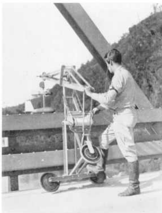
Figure 2. Equipment Used in Making Discharge Measurements from Bridge
