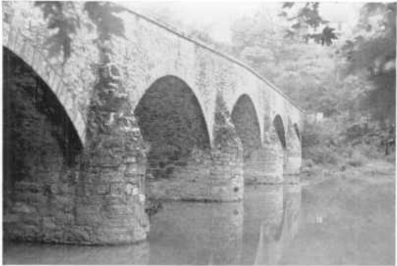
PLATE 18, Figure 1. Old Road Bridge at Wilson, Conococheague Creek. Masonry largely Stones River and Beckmantown limestone.
