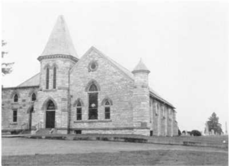
Figure 2. St. Pauls Church on U. S. 40 between Conococheague Creek and Clear Spring. Mostly Stones River and Beckmantown limestones.
