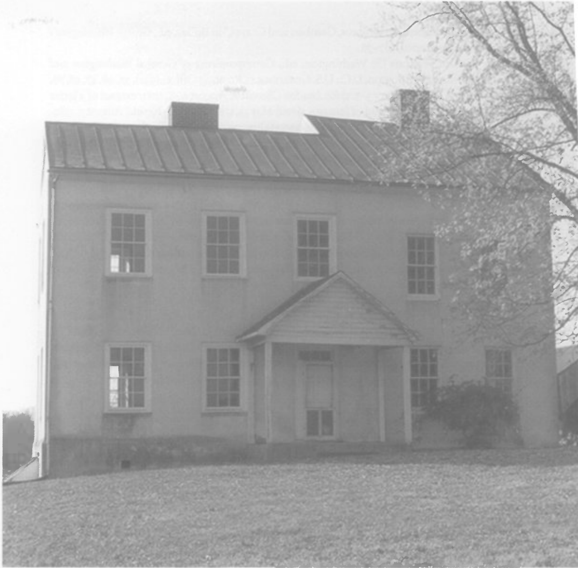
East elevation of the main house at l'Hermitage. The left portion was constructed in 1794, the taller right section about 1820. Embedded within the structure is a smaller building that was already standing when the Vincendieres established residence on the property in early 1794. (Author's photograph.)
