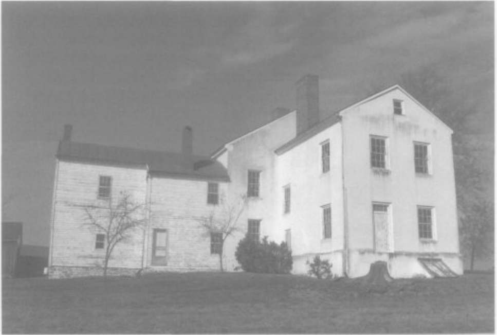
Northeast view of the main house. To the right is the 1794 "east wing." Behind it is the c.1820 addition. Wooden sections include an eighteenth-century one-story log kitchen at far left and next to it a later frame infill dating from the third quarter of the nineteenth century. (Author's photograph.)
