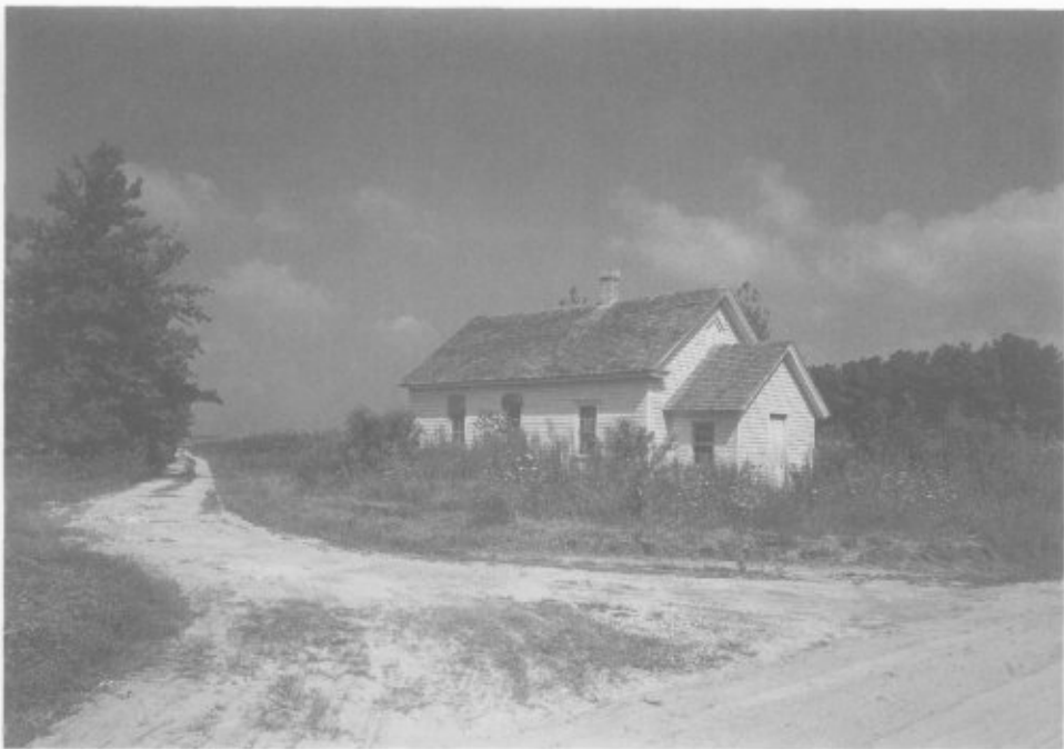
White School House, Caroline County, no date.
