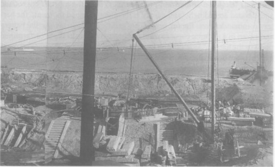
Artillery emplacements under construction at Hawkins Point, November 30, 1897. (National Archives.)
