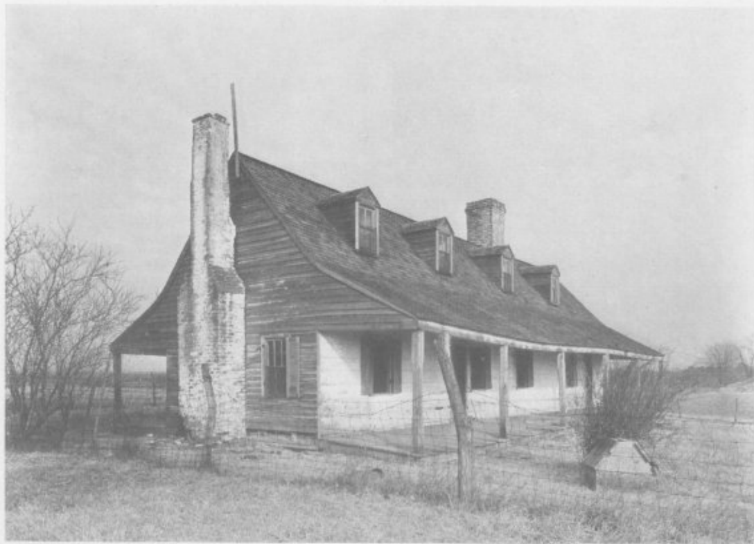
West view of "Susquehanna," before removal, showing partly free-standing chimney. Photo by Edison Institute, Dearborn, Mich. Courtesy Maryland Room, Pratt Library.
