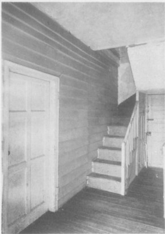
Passage and main stair of "Susquehanna." Wall at left is of ordinary weatherboarding. H. A. B. S. photo.
