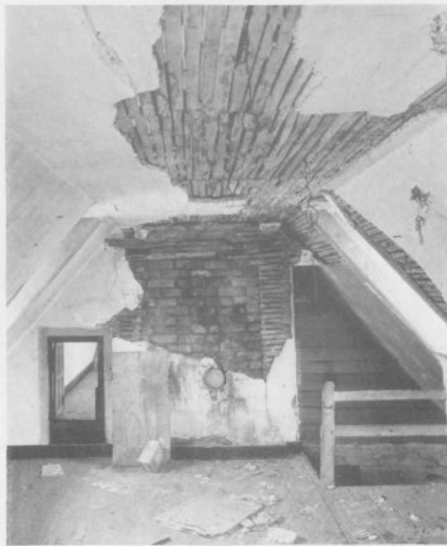
Room over kitchen, showing steep stair from lower floor, tiny door to next room, and hand-hewn lathes. H. A. B. S. photo.
