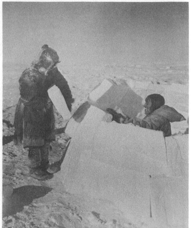
Igloo Building - An art which is rapidly disappearing in the Far North.
