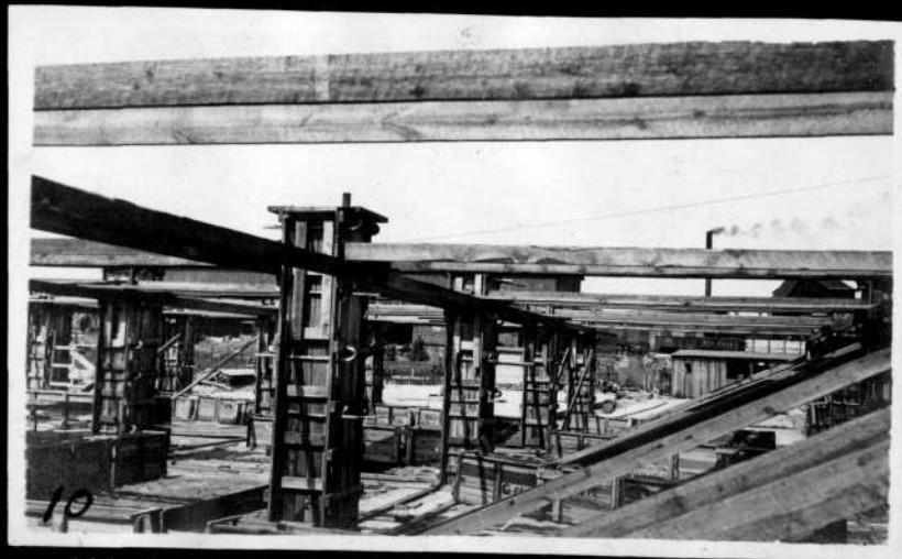
10 Werk Soap Co. Showing method of ledgering col. forms.
