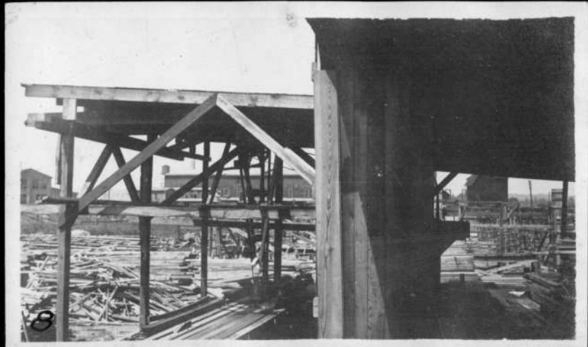
Werk Soap Co.. View of swing arm or cut off saw
