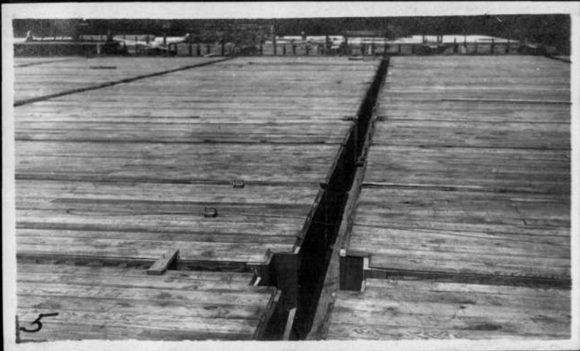
Werk Soap Co.. Forms assembled ready for placing of steel.
