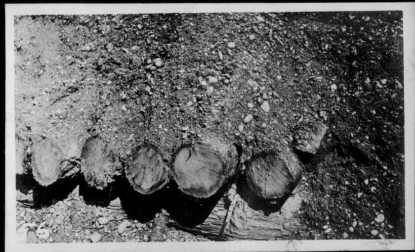
Remains of a buried bridge across stream at Charles St Ave
