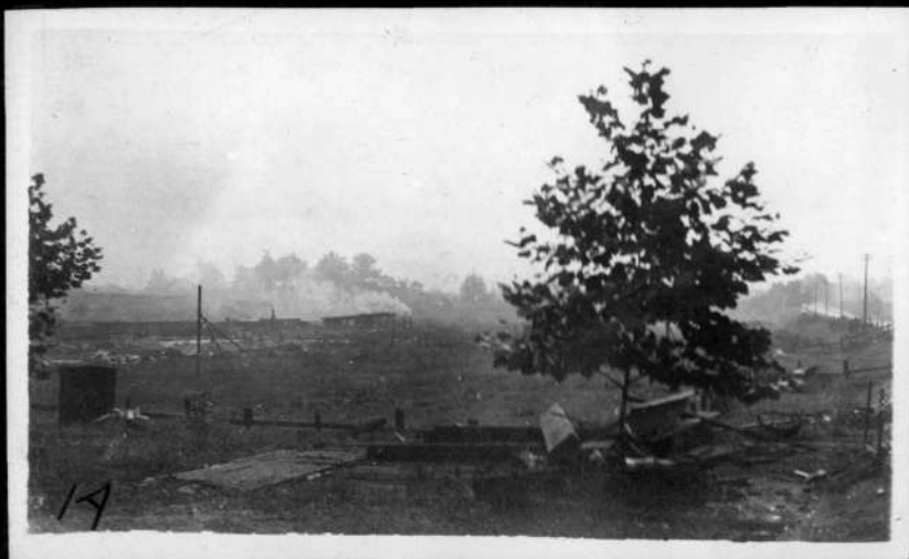
Werk Soap Co. Looking across the site from the ice plant.
