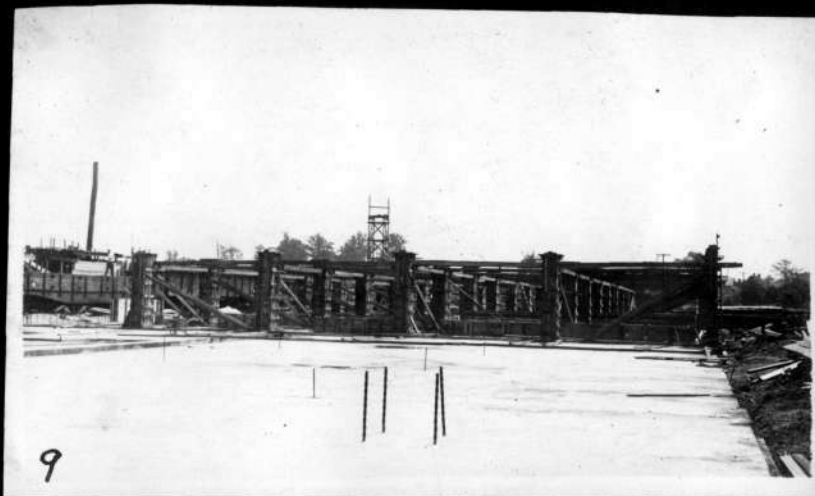
9 Werk Soap Co. Col. forms erected and ready for beams and girders. First section of South Building.
