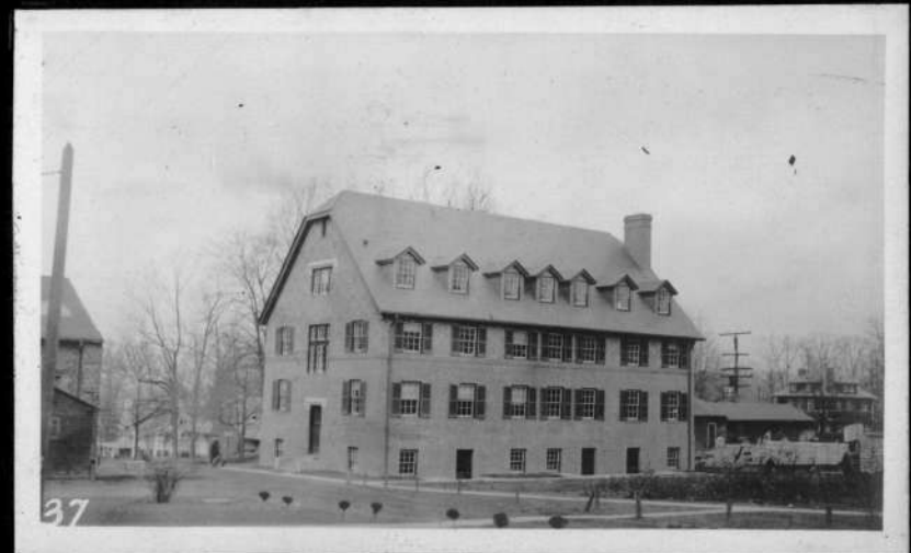
Office Building Roland Park
