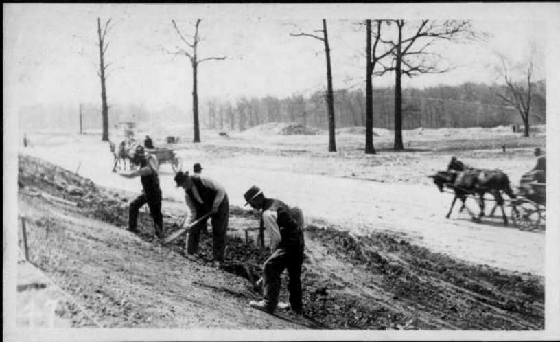
Grading Greensy sides near Woodover Road.
