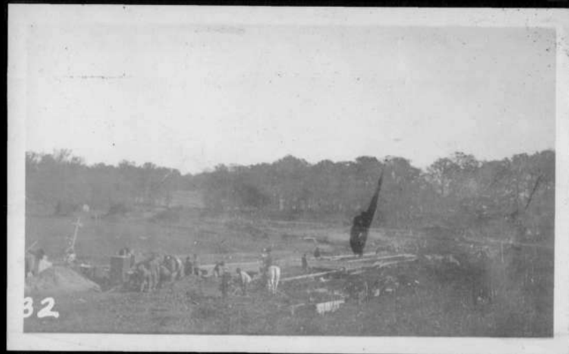
Southerly junction of St. Paul and Greenway
