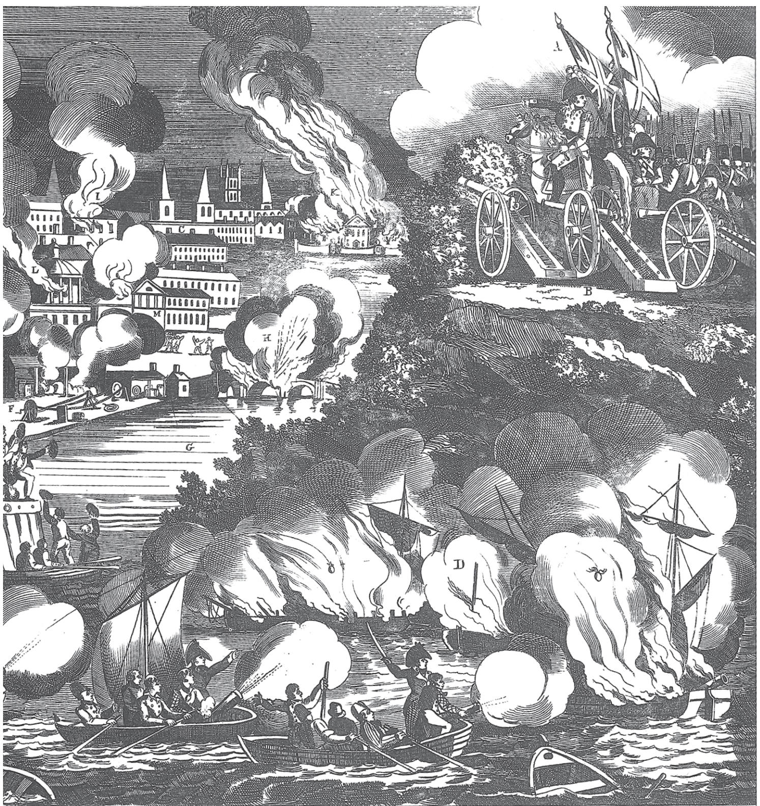
CAPITAL OF THE UNITED STATES OF AMERICA WAS TAKEN BY THE BRITISH FORCES UNDER MAJOR GEN L ROSS and their Dock Yard with a Frigate and a Sloop of War Rope-walk Arsenal Senate House Presidents Palace War Office Treasury and the Great Bridge to thirty Million of Dollars. Published Oct 11. 1814. by G. Thompson, N o 43 Long Lane West, Smithfield.
