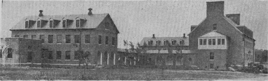
Front view of new hospital at Crownsville, Md., for feeble-minded colored children.
