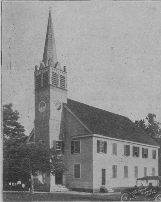
Shiloh church, Northumberland County. This church in the open country has over 1,100 members
