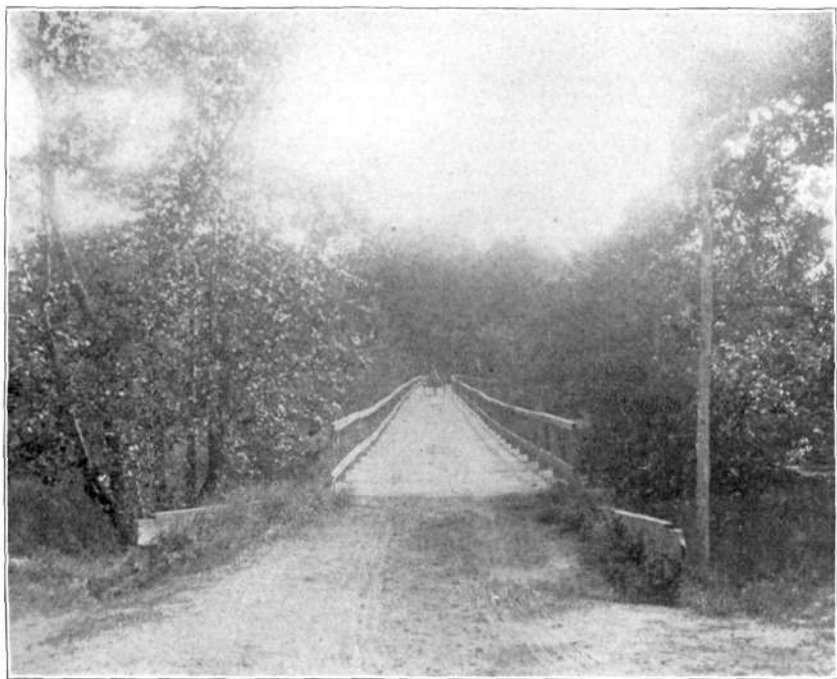
Bridge Over the Nottoway River at Jerusalem.
