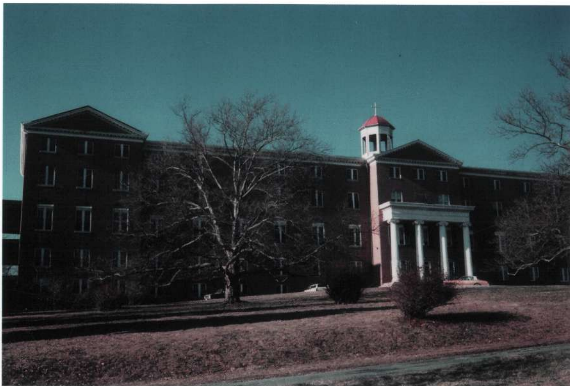
Plate 19. Mount de Sales Academy of the Visitation, Catonsville, Maryland
