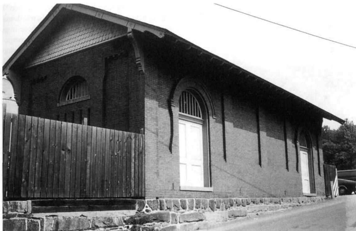
Fig. 40. B&O Freight House, Ellicott City, Maryland
