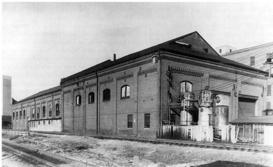
Fig. 39. Belt Railroad Powerhouse, Baltimore. Smithsonian Institution, Transportation Collection
