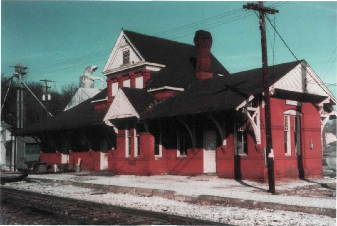
Plate 2. B&O Station, Sykesville, Maryland
