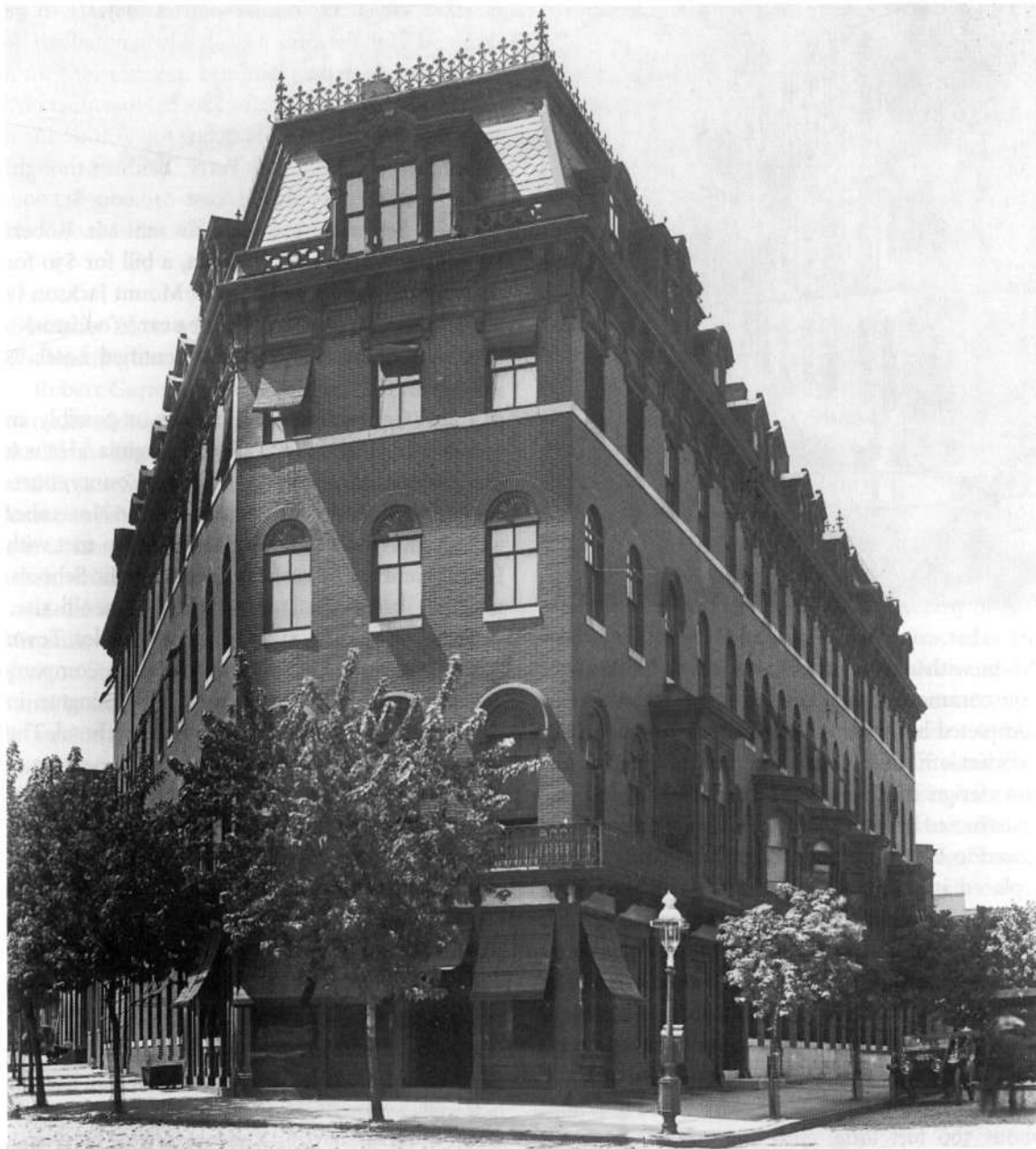
Fig. 81. Albion Hotel, Baltimore. The Maryland Historical Society, Baltimore, Maryland
