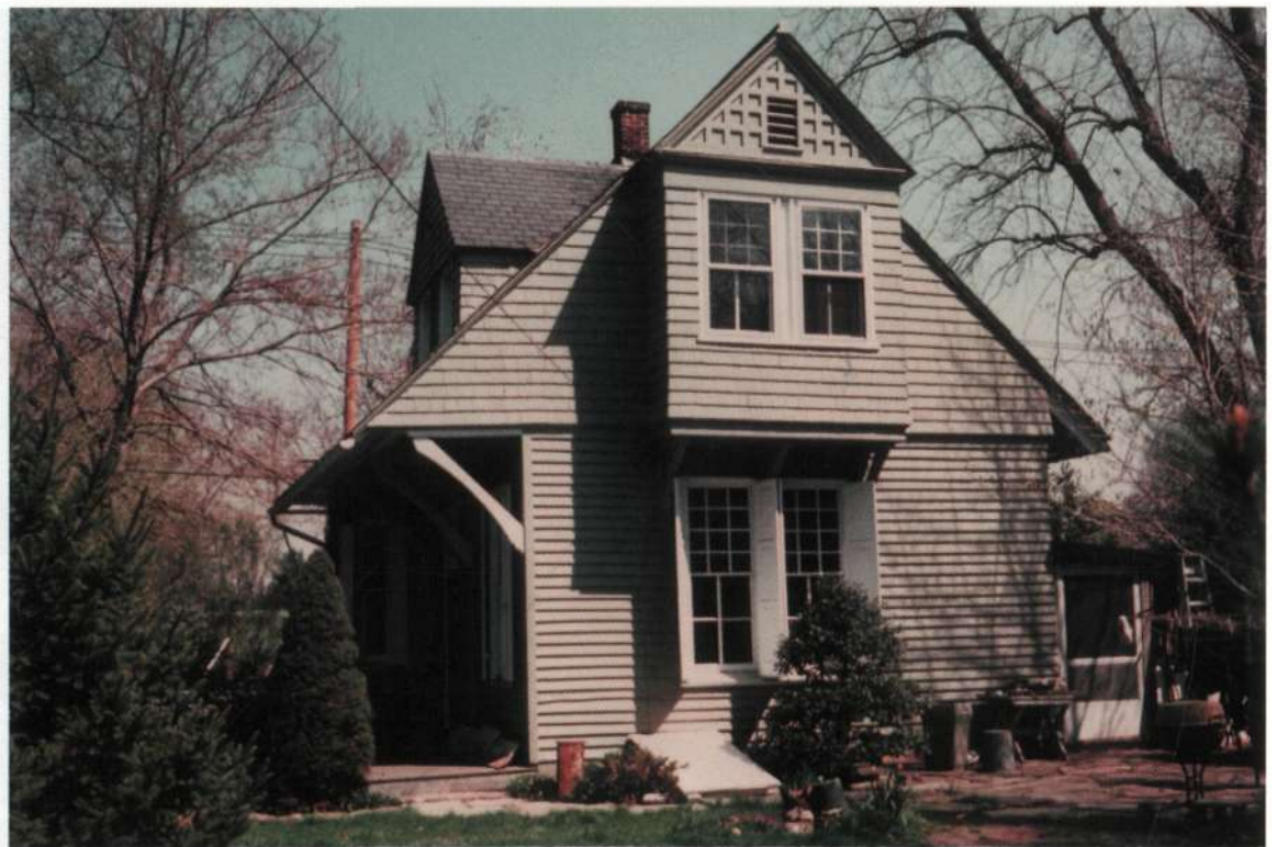
Plate 8. Homeland Station, Lake Avenue
