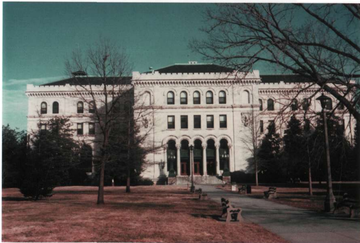
Plate 22. Mess Hall (Grant Building), USSH, Washington, D.C.
