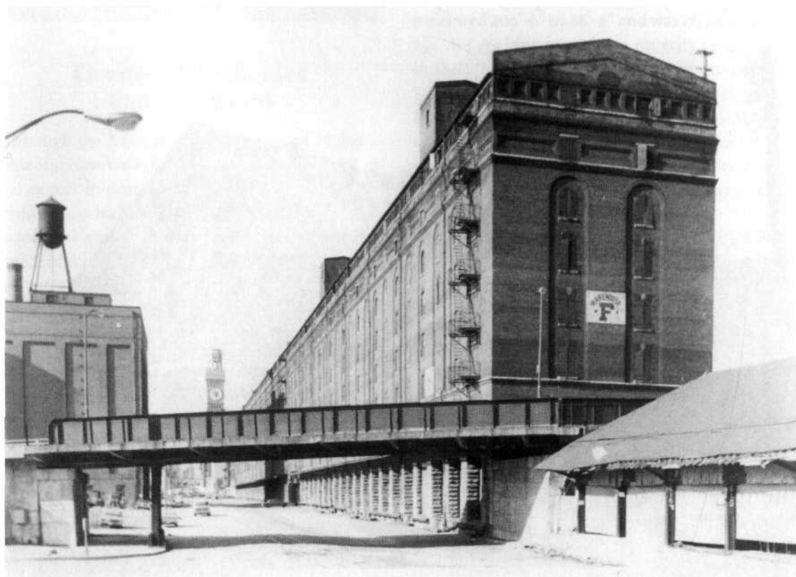
Fig. 44. Camden Station Warehouse, Baltimore. Smithsonian Institution, Transportation Collection
