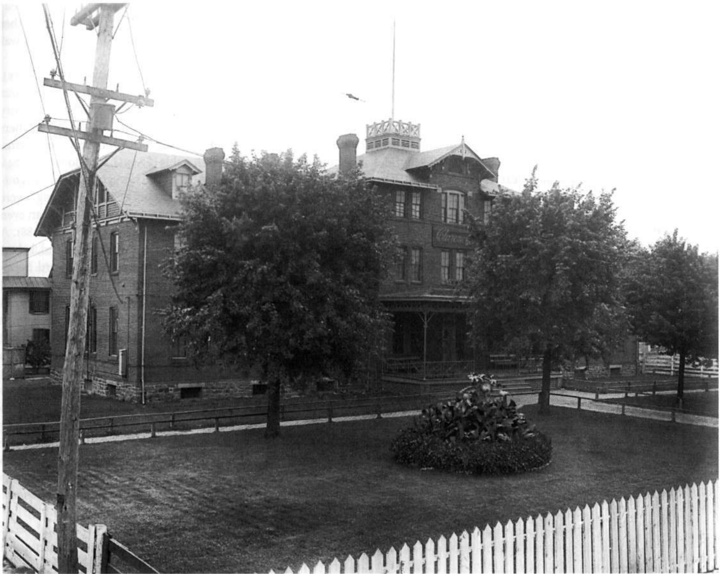
Fig. 45. Claremont Hotel, Baltimore. Photography Collections, University of Maryland, Baltimore County
