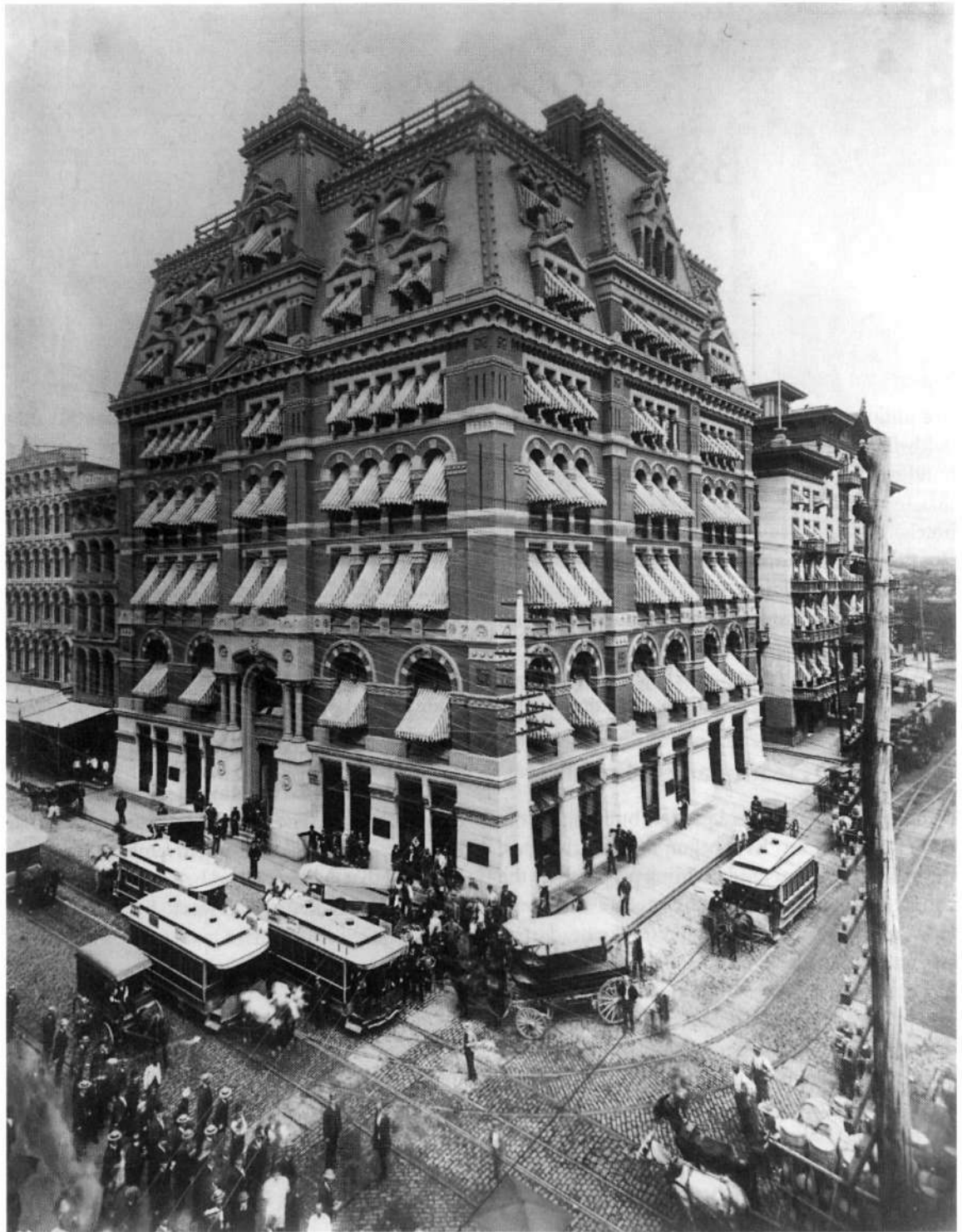
Fig. 34. B&O "Central Building," Baltimore. The Maryland Historical Society, Baltimore, Maryland
