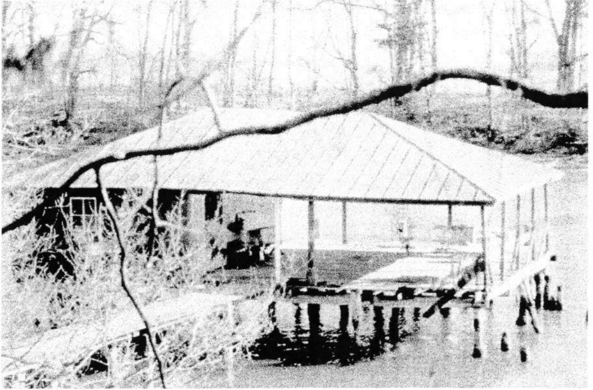
POPLAR GROVE BOATHOUSE
