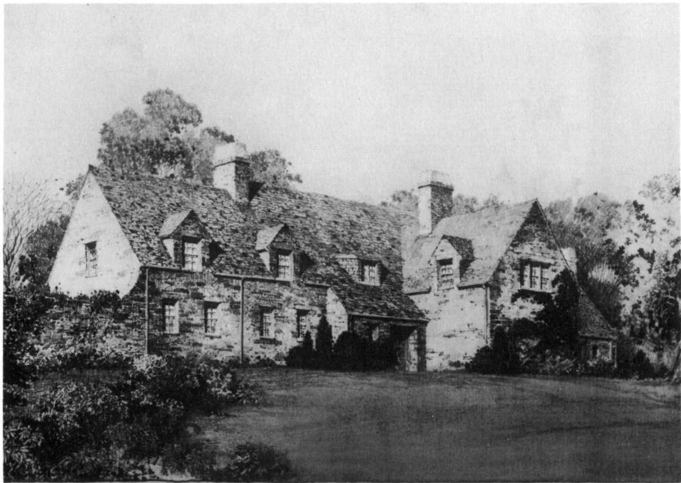
The "Poplars", located at Poplar Hill. Due to the impossibility of securing a good photograph of the actual building (which faces north) the above reproduction was made from the architectural rendering.
