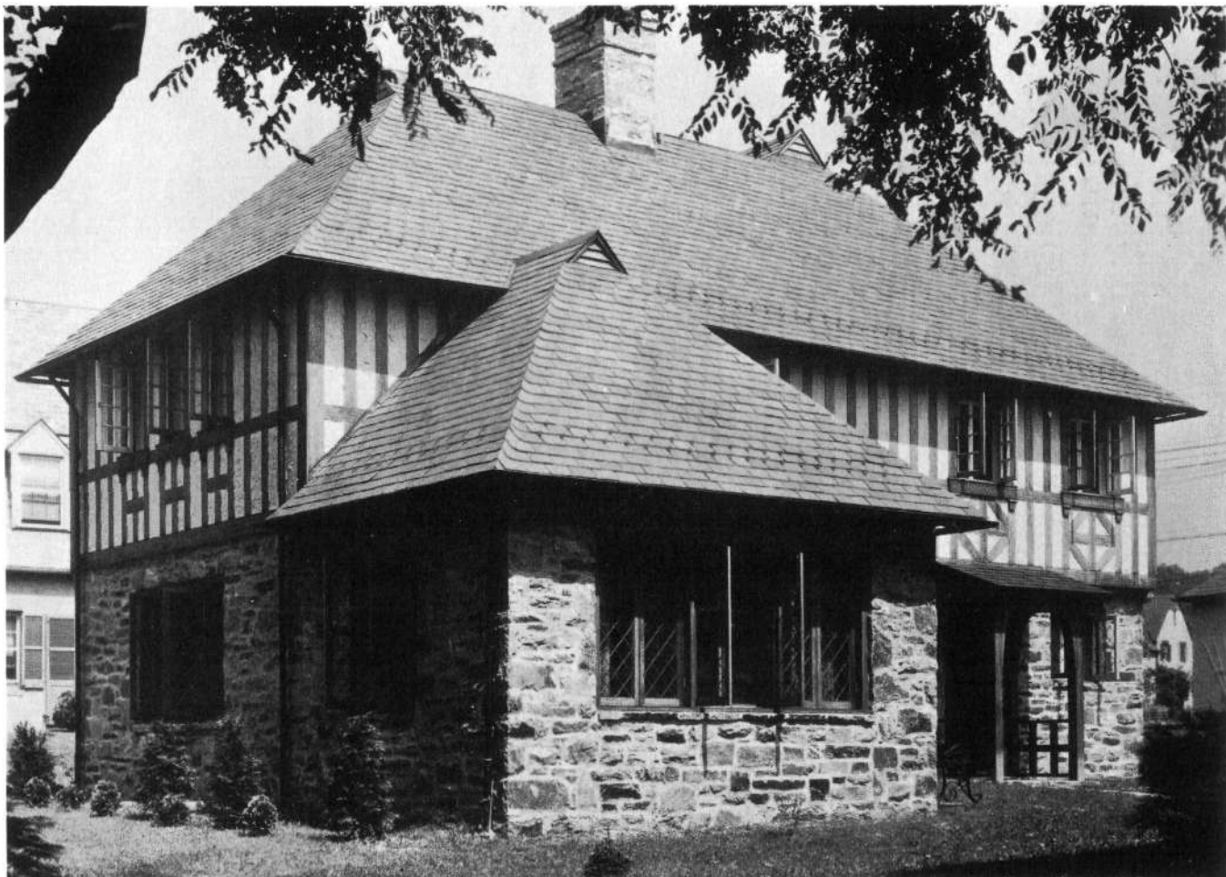
Residence of Mr. and Mrs. Albert E. Heimert on St. Dunstan's Road, Homeland, Baltimore. View from east.
