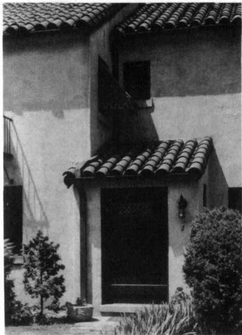
D ETAIL showing the entrance door and texture of stucco residence of Mr. and Mrs. Frederick Arnold Kummer, Guilford, Baltimore.
