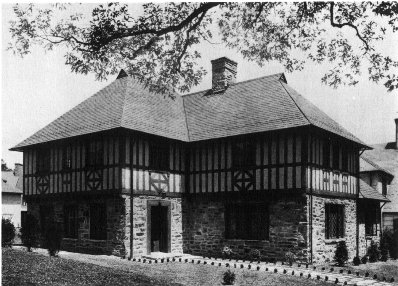
The residence of Mr. and Mrs. Albert E. Heimert on St. Dunstan's Road, at Homewood.
