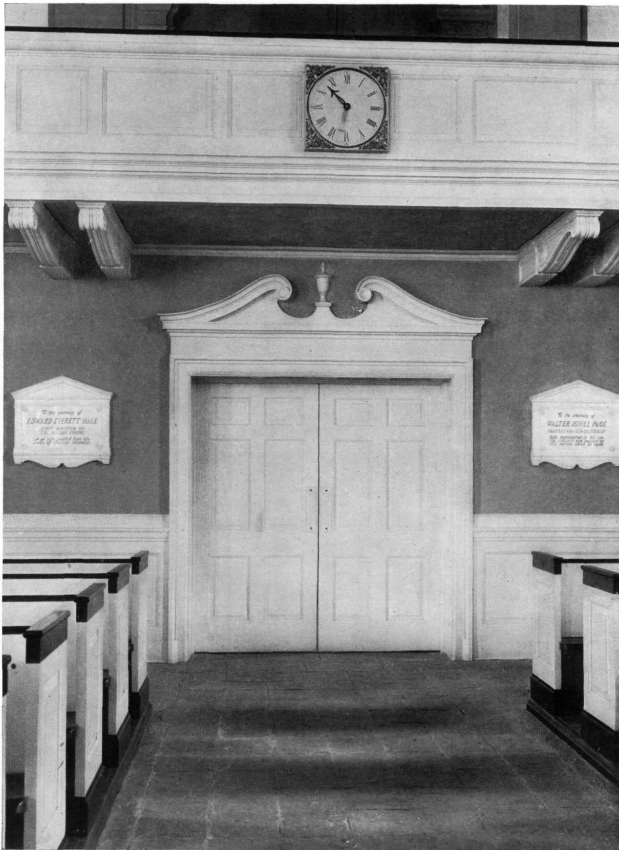
MAIN VESTIBULE DOORWAY, THE VILLAGE CHAPEL, PINEHURST, N. C. HOBART B. UPJOHN, ARCHITECT
