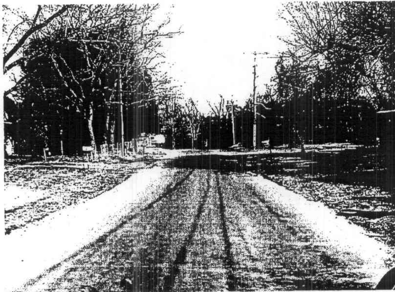
Looking Westerly Along Pier Street
