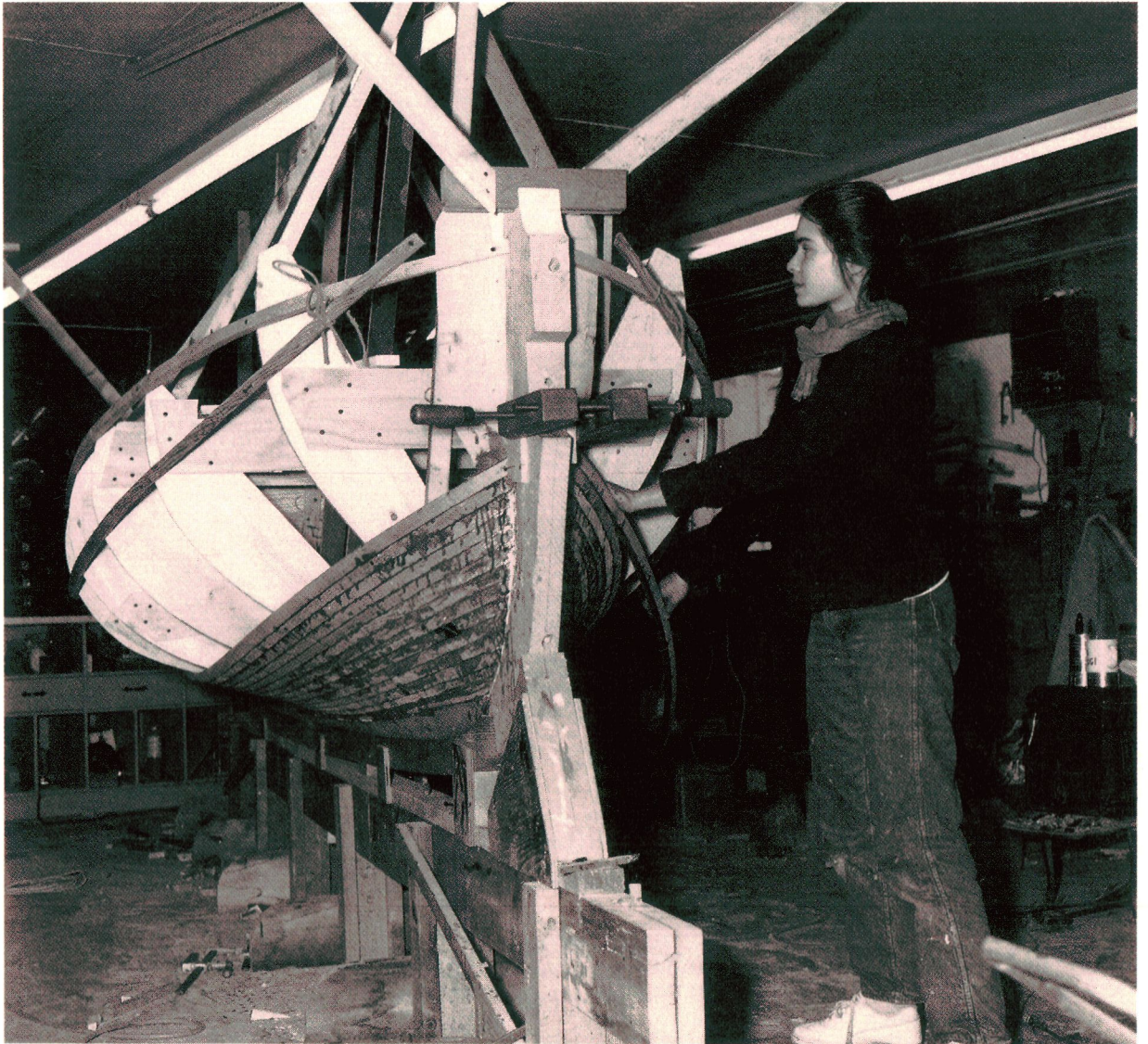
Laurie Rawl, daughter of builder Allen Rawl, secures a plank to the Maryland Federalist . Photo: Paul Houston, courtesy Maryland Federalist Foundation.
